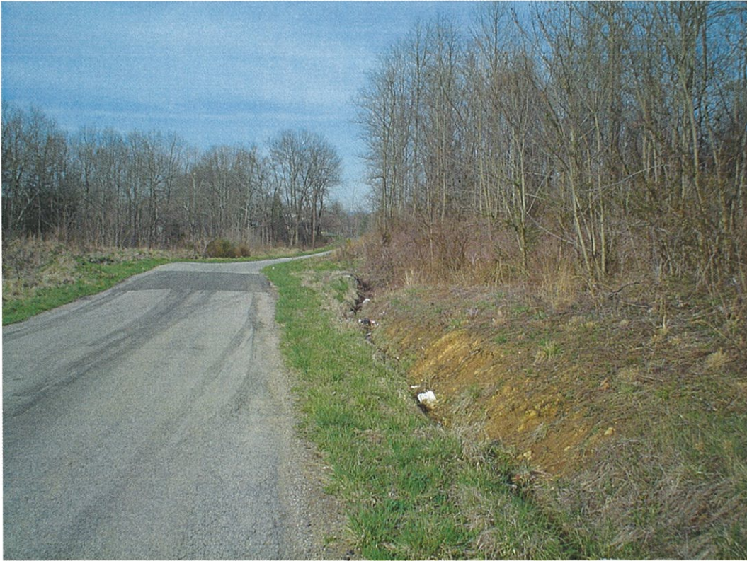
Looking West at Morris Lane at Bridge Location
