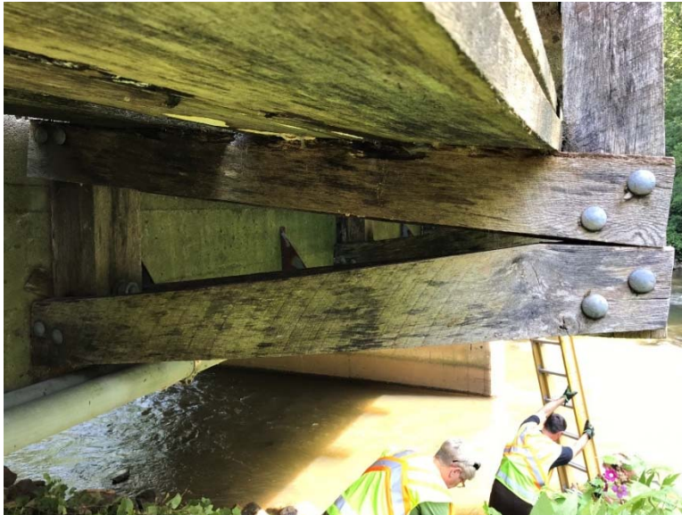
Picture # 1 - Typical downstream sidewalk cantilever support.
