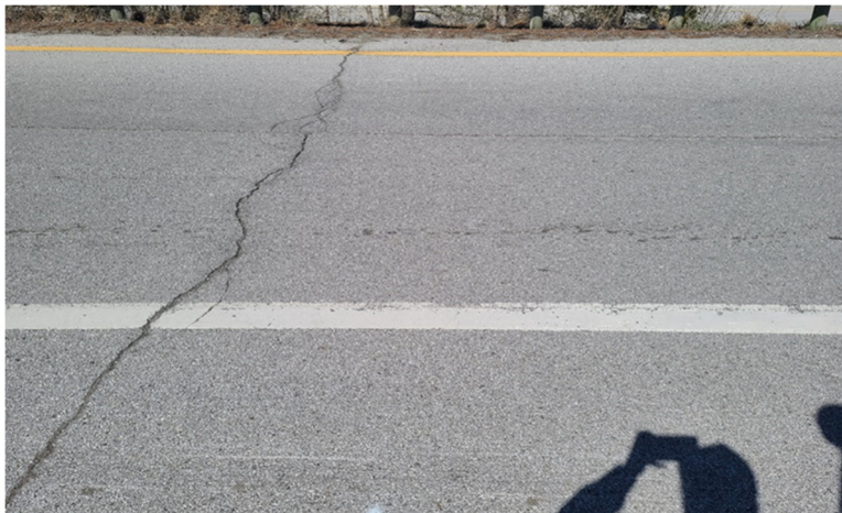
Photograph 8: Pavement Condition Along Ramp 12
