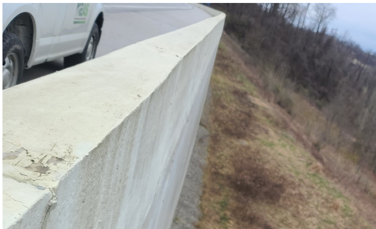
Photograph 5: Retaining Wall Supporting IR-70 Roadway Sidehill Fill
