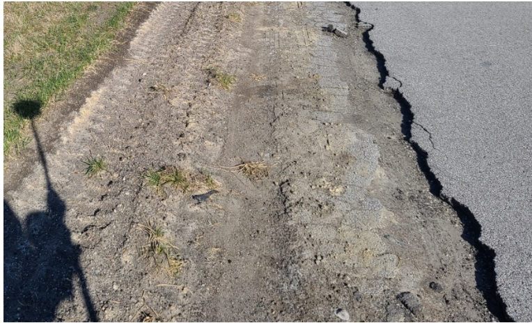
Photograph 2: IR-70 Pavement Transverse Cracking
