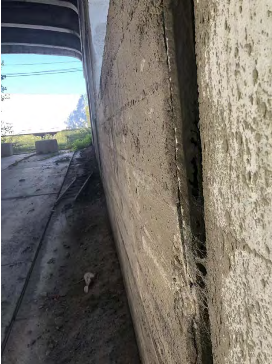
P9: Titled retaining wall at Bent 47
