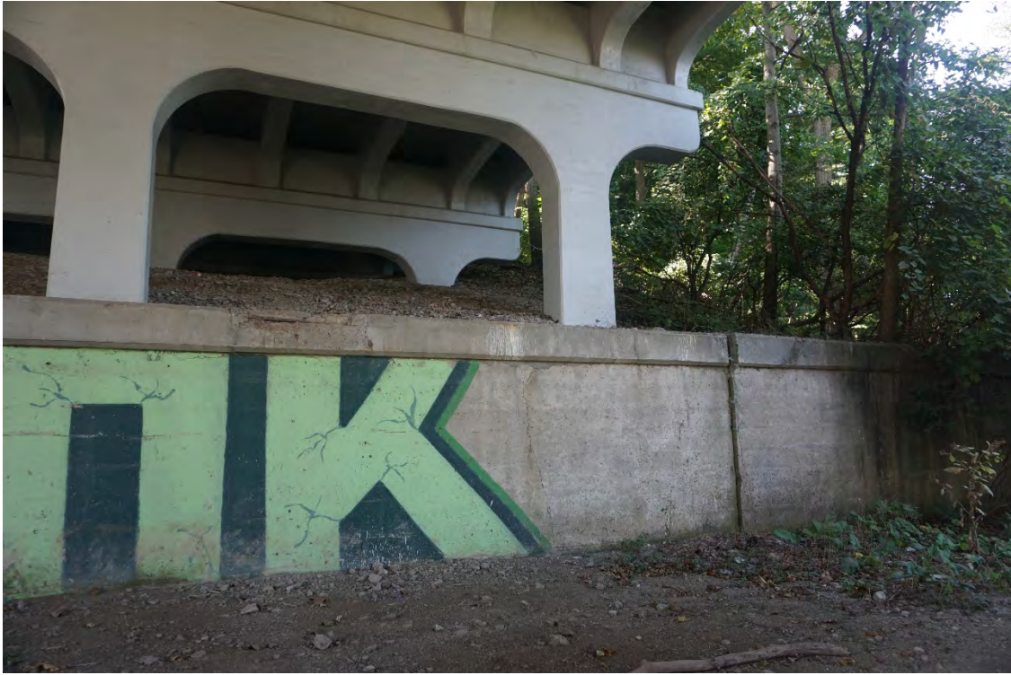
P6: Tilted shoring and concrete spalling at the forward abutment along SR 14
