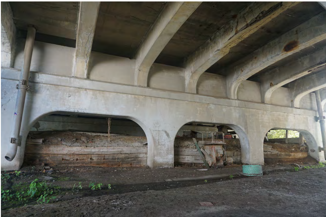
P6: Tilted shoring and concrete spalling at the forward abutment along SR 14
