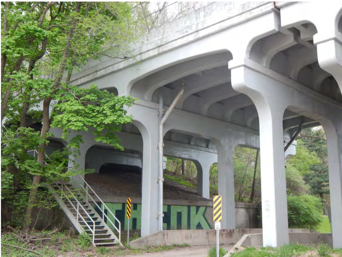
View of Stairs and Henry Street Bridge over Mill Creek Culvert
