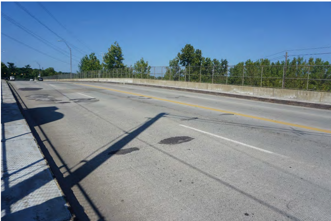
P13: Pavement condition on the bridge
