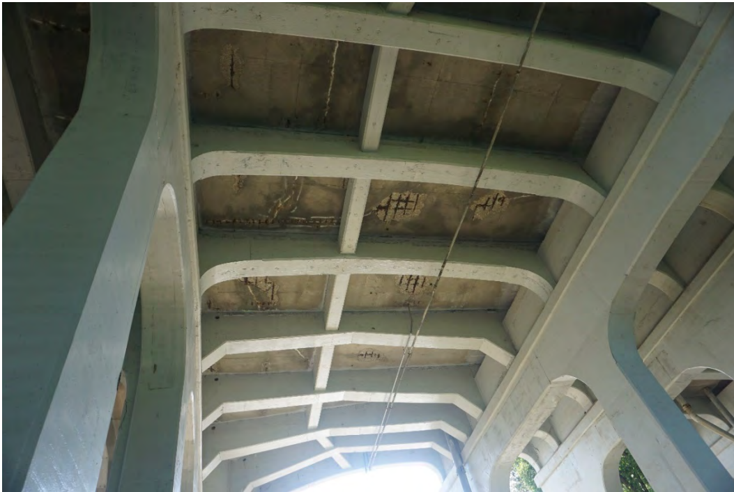
P11: Concrete spalling under the bridge deck
