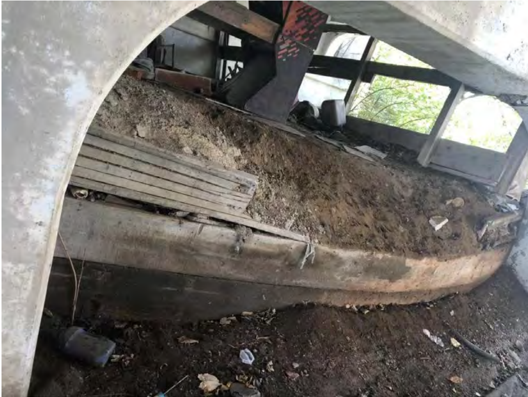
P11: Concrete spalling under the bridge deck
