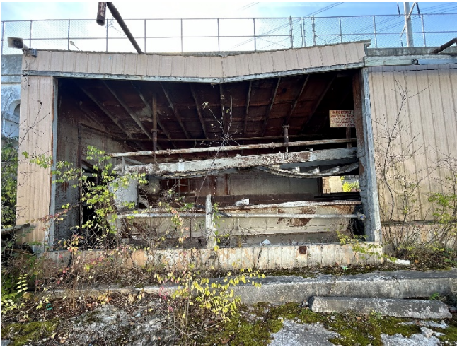
View of the entrance to the building.
