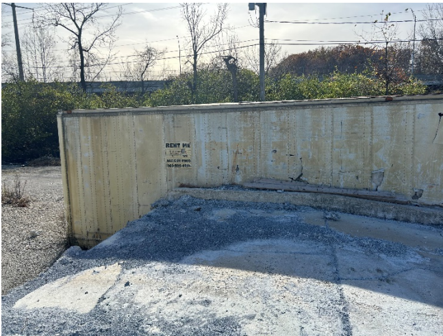
View of the northern side of the trailer.
