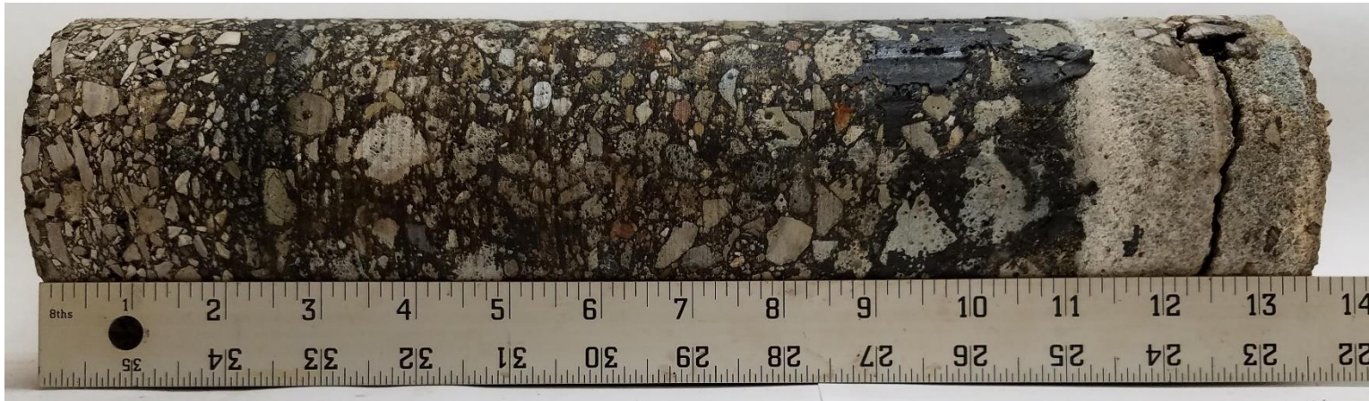
C-14 (11 1/4" Asphalt Concrete, 2 1/4" Concrete)
