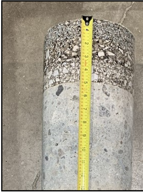
Coring No. B-012-0-20 Total Length: 14.000" Location: U.S. 422 W entrance ramp STA 442+67 3' RT
