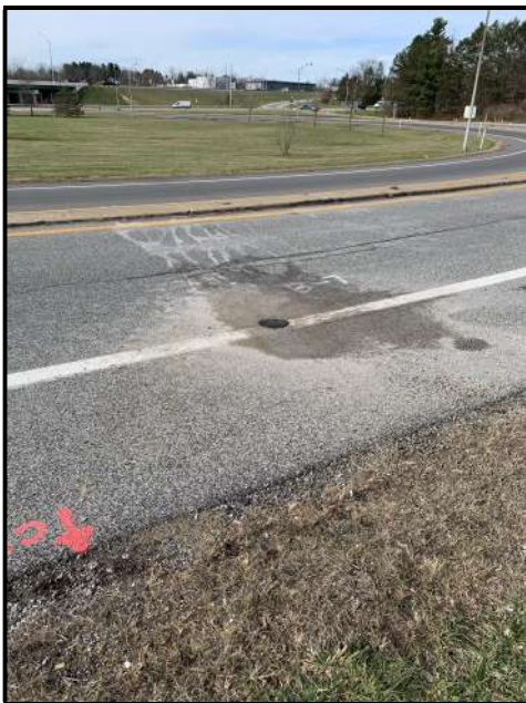
Boring No. B-014-0-20 Elevation: 1067.5 Location: U.S. 422 W exit ramp STA 650+11 22' RT
