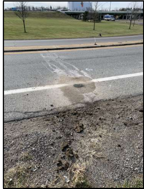
Boring No. B-013-0-20 Elevation: 1065.2 Location: U.S. 422 W exit ramp STA 647+58 1' RT
