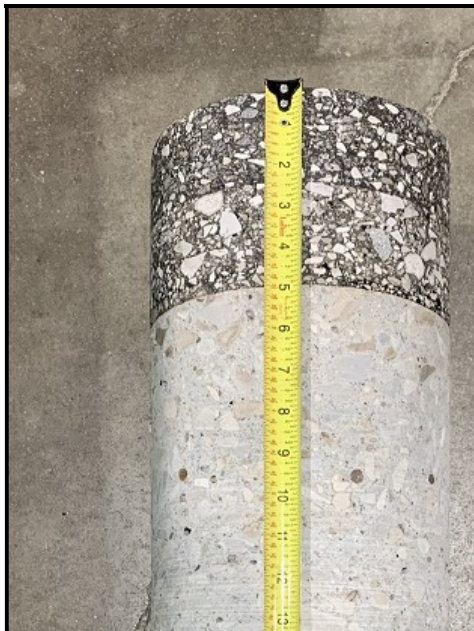
Coring No. B-010-0-20 Total Length: 14.500" Location: Harper Rd southbound left turn lanes STA 73+46 4' LT
