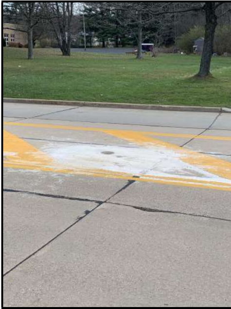
Boring No. B-001-0-20 Elevation: 1072.6 Location: Harper Rd center striped zone STA 58+38 5' RT
