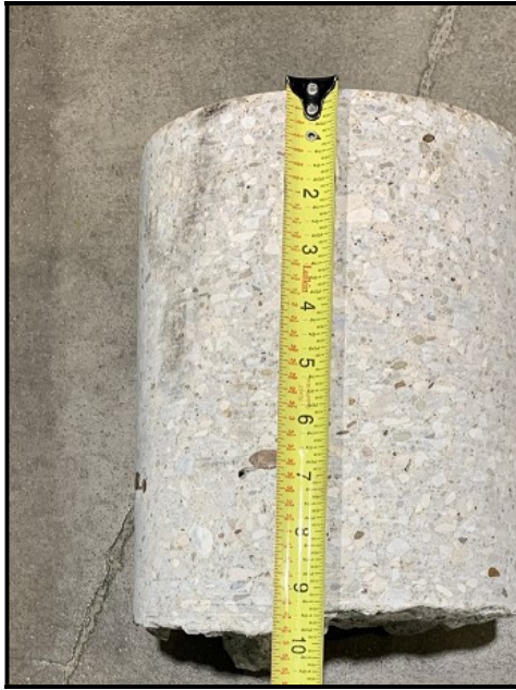
Coring No. B-001-0-20 Total Length: 9.750" Location: Harper Rd center striped zone STA 58+38 5' RT
