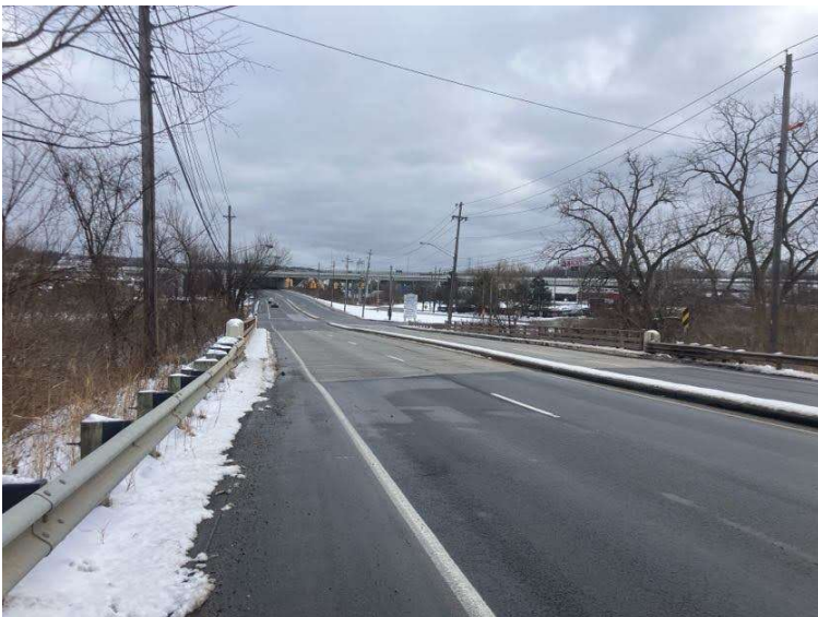
PHOTO 1 View of bridge CUY-17-14.14, facing east.
