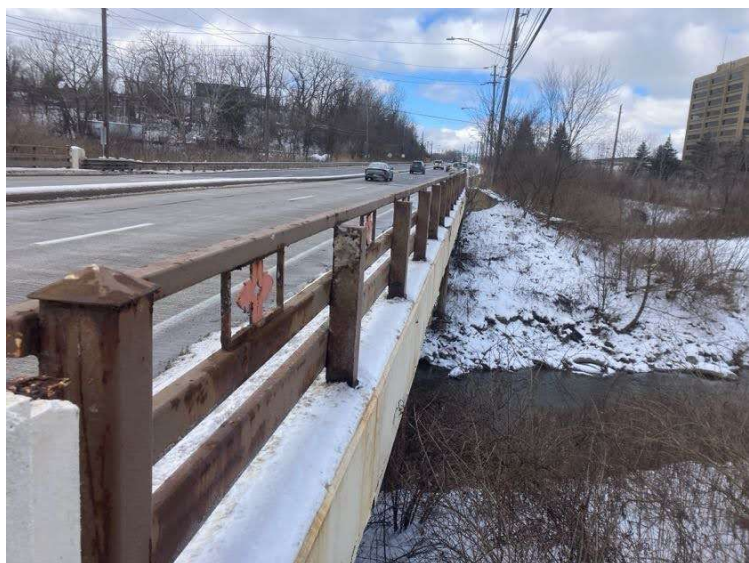
PHOTO 3 View of the north side of the structure. No utilities were affixed to the structure.
