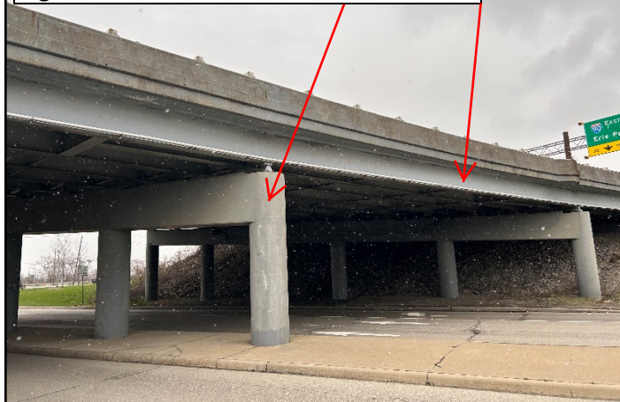
Figure 6: View of Paint on Concrete & Steel
