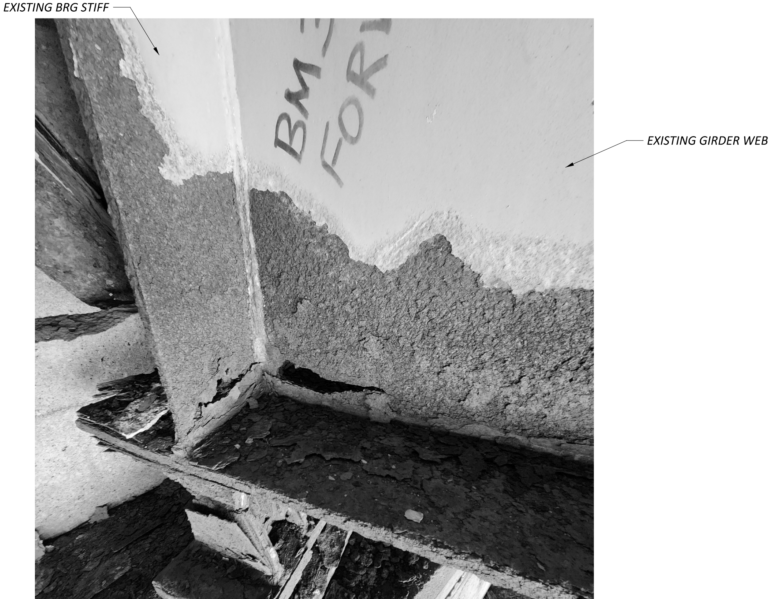
REPAIR LOCATION INSPECTION PHOTO GIRDER 3 AT EAST ABUTMENT
