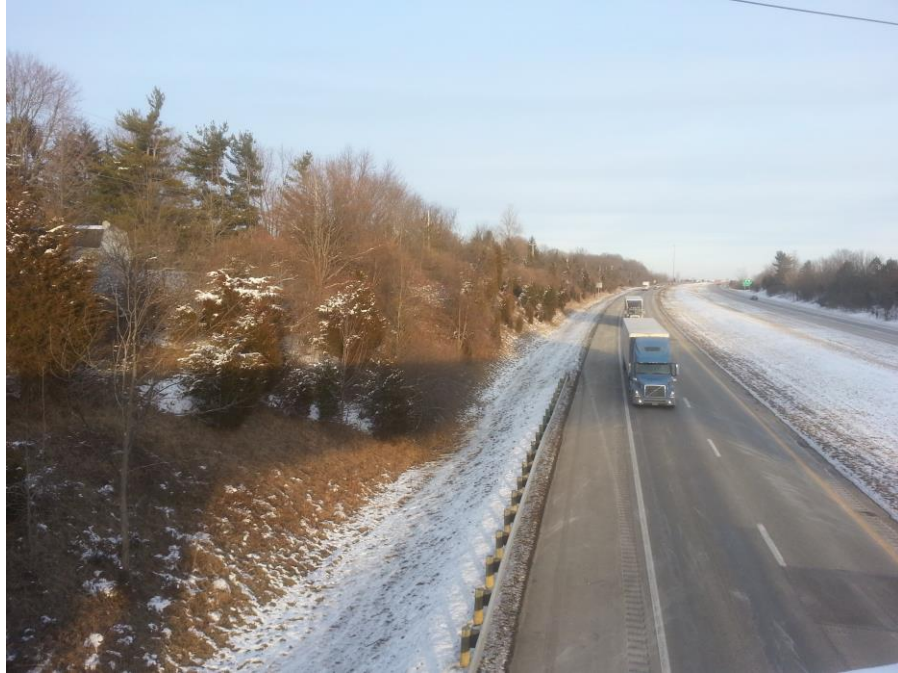
Photograph 1: View of the proposed wall site looking east from the Lambert Rd overpass.
