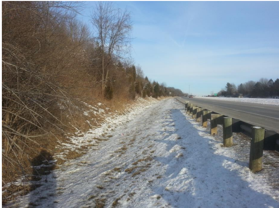
Photograph 2: View of slope at the western end of the wall.
