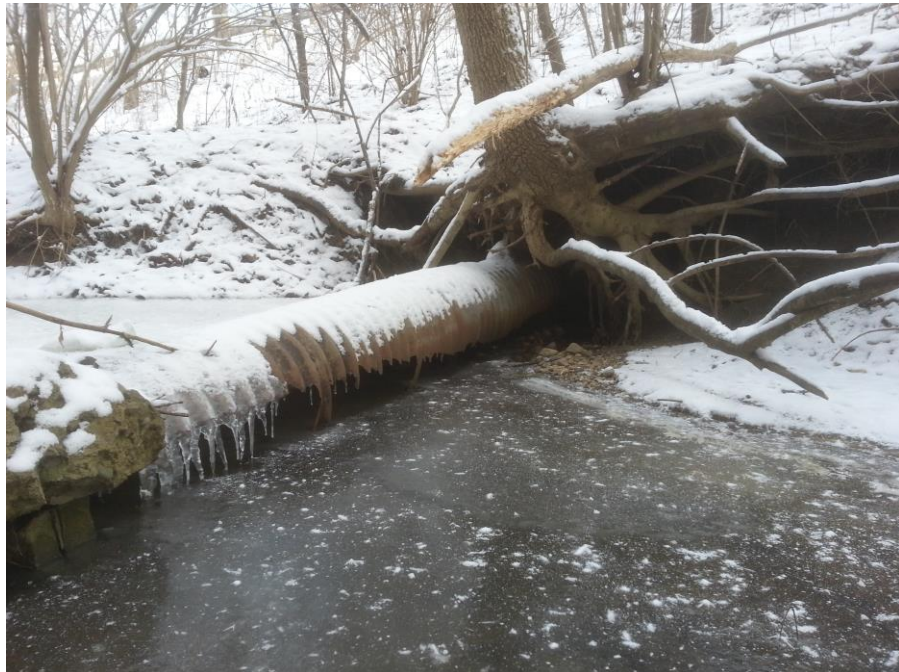
Photograph 6: Culvert beneath IR-71.
