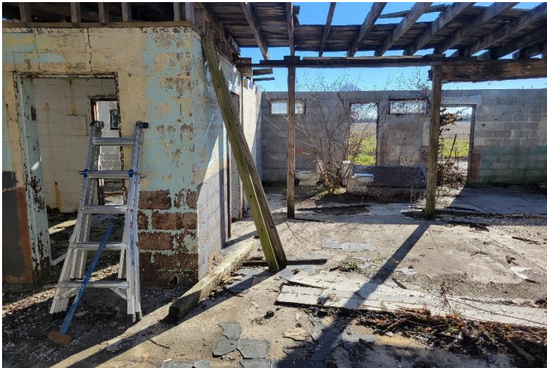
Photo 3 – View of central area of concrete structure looking south.
