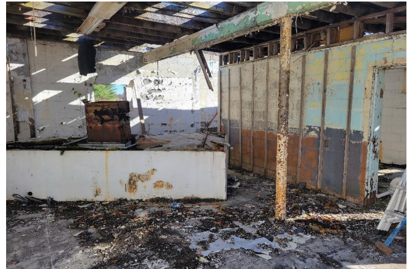
Photo 4 – View of central area of concrete structure looking northeast.
