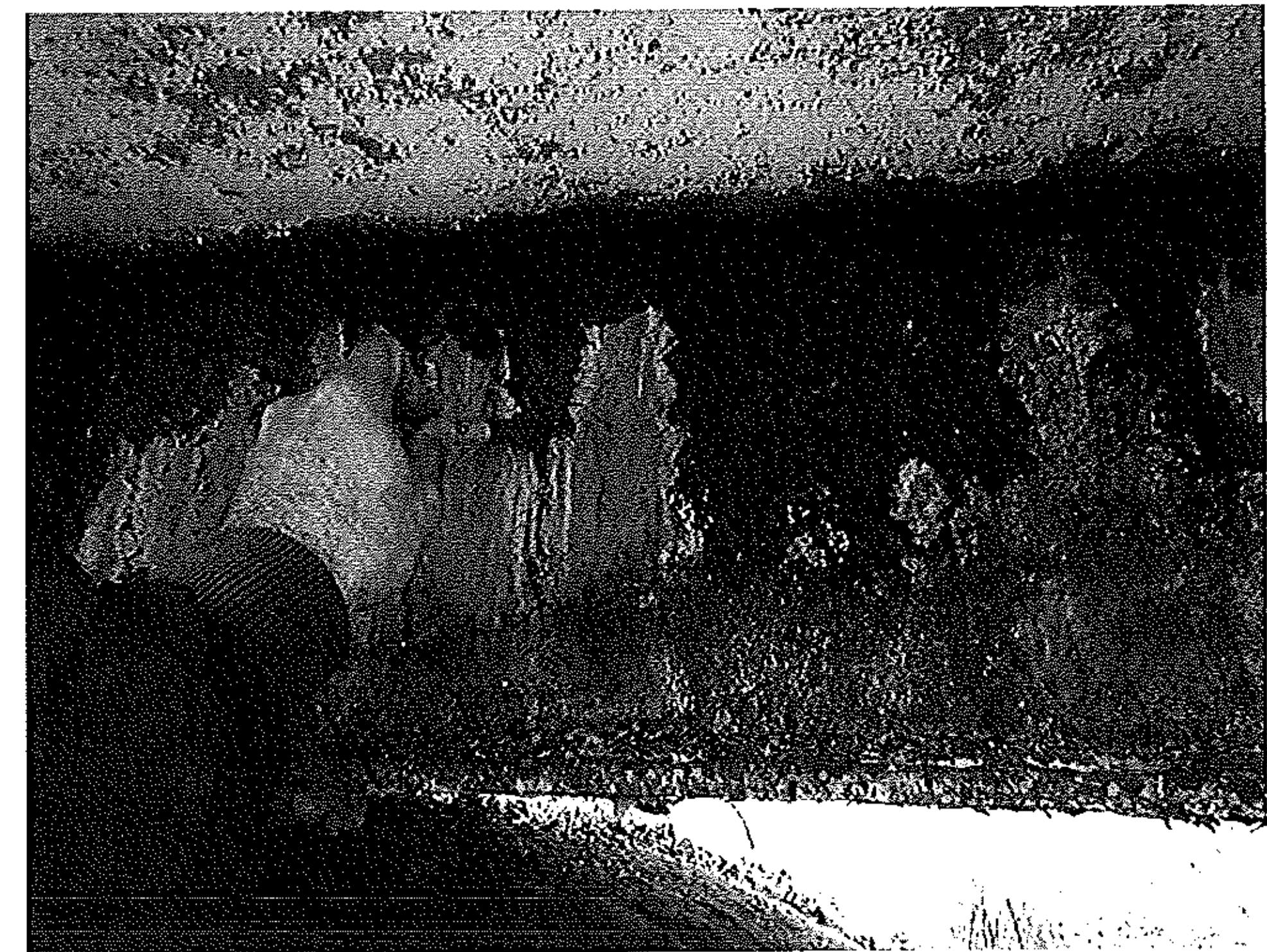
Photograph 10. View of steel girder paint flakes (Sample S2), from the northern side of the bridge.
