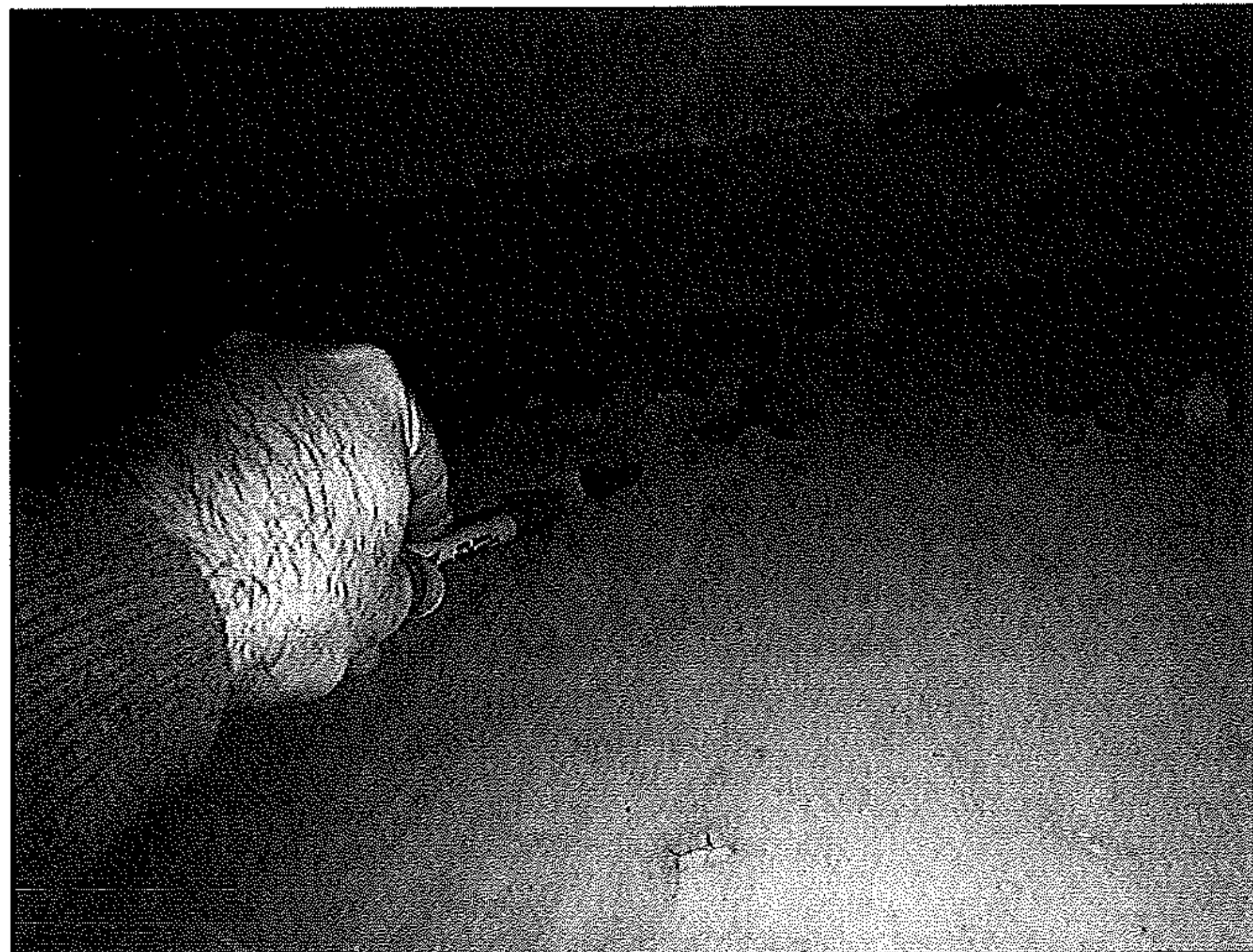
Photograph 8. View of steel girder paint flakes (Sample S1), from the northern side of the bridge.
