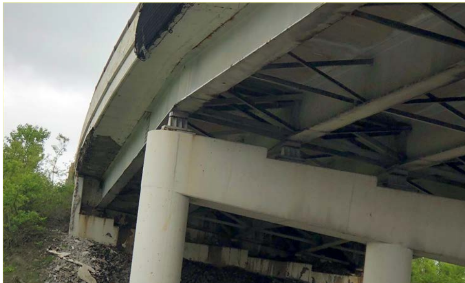
Photograph 2: Spalling and Exposed Rebar at Bridge Deck Ends
