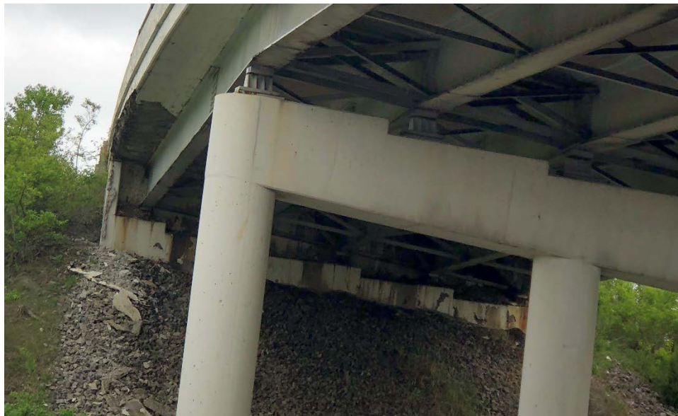
Photograph 4: Spill-Through Slope at Rear Abutment
