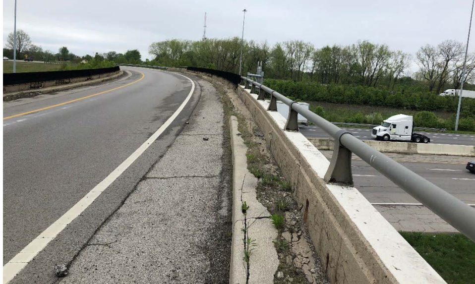
Photograph 2: Spalling and Exposed Rebar at Bridge Deck Ends
