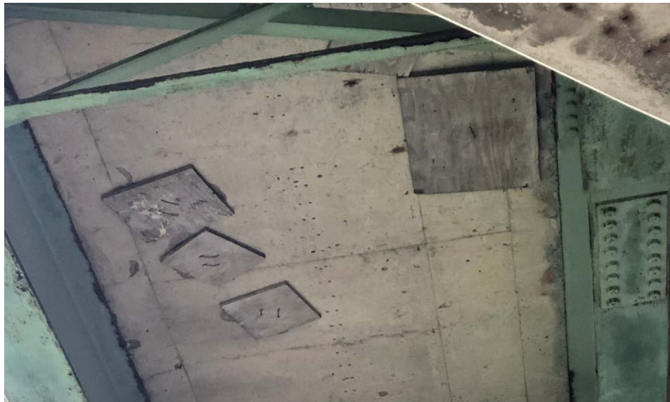
Photograph 2: Signs of Patching in Underside of Bridge Deck
