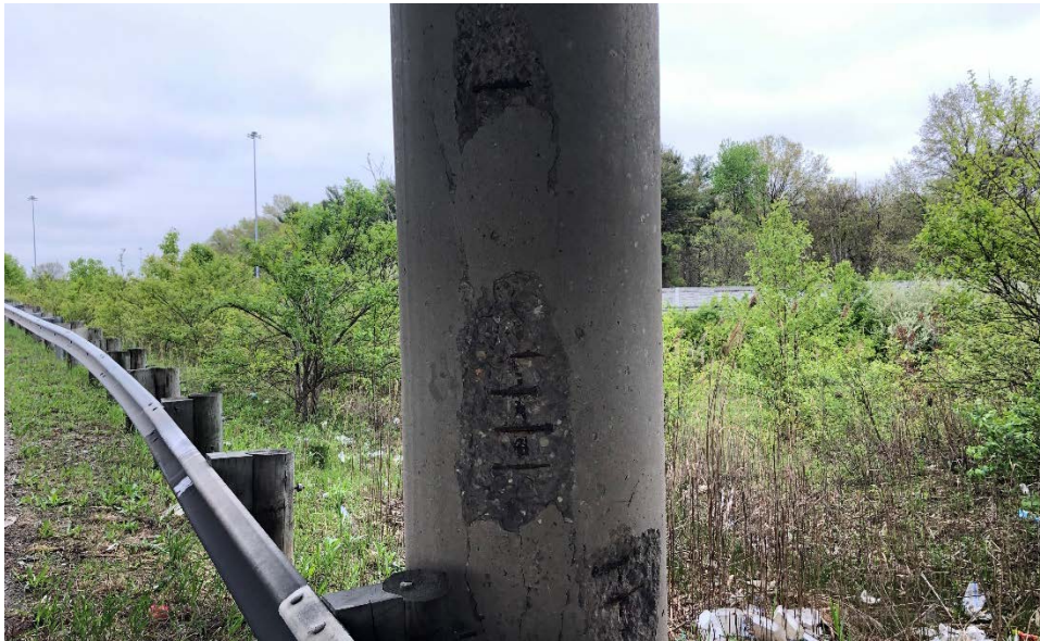
Photograph 4: Spalling and Exposed Rebar at Eastern Pier
