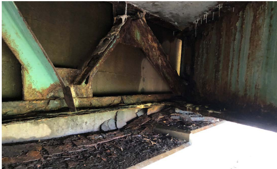
Photograph 2: Signs of Patching in Underside of Bridge Deck
