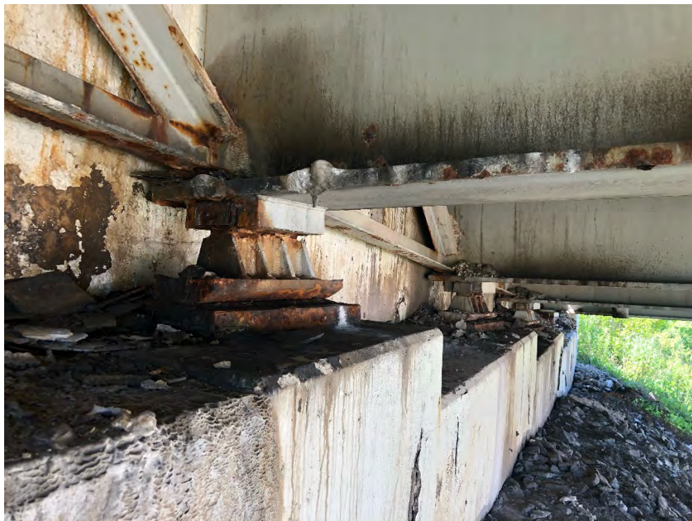
Photo 8: Rocker plates on Bridge 28.31.
