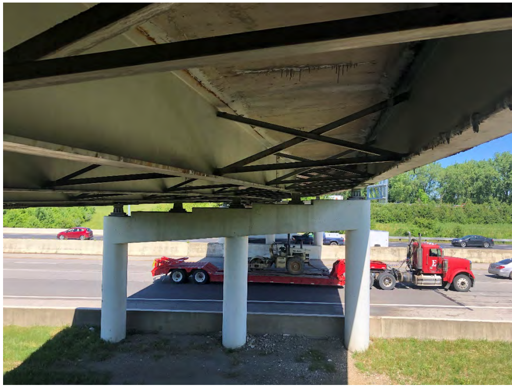
Photo 7: Underside of Bridge 28.31, concrete deck and steel beams with concrete piers.
