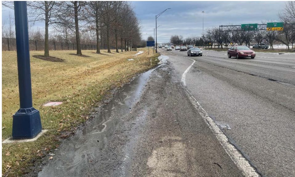
Photograph 6: Standing water at Edge of Easton Way
