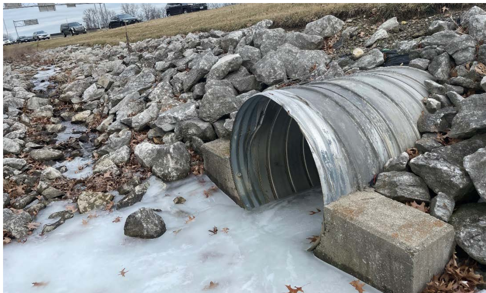
Photograph 3: Flexible Pipe Culvert
