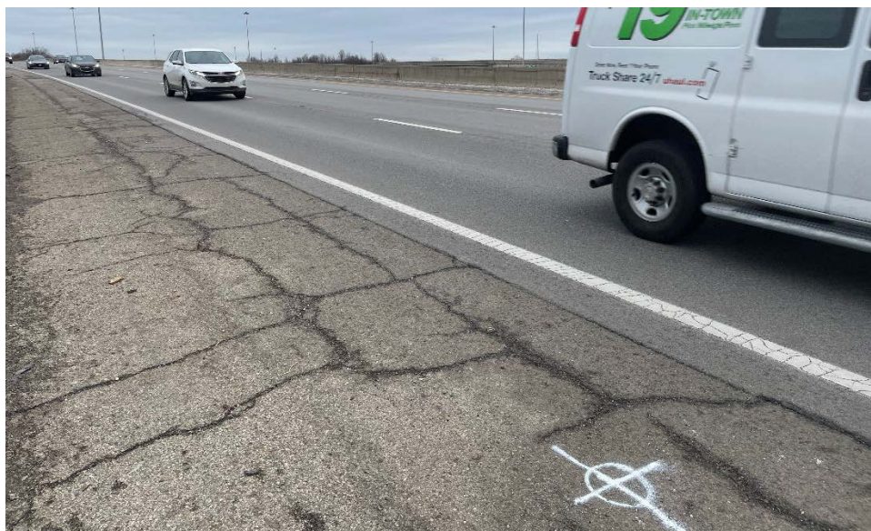
Photograph 1: Overall Pavement Condition of IR-270 SB Exit Ramp to Easton Way
