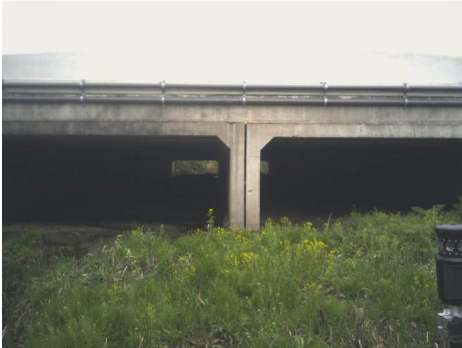
Figure 3. Existing Culvert Outlet End (looking upstream)
