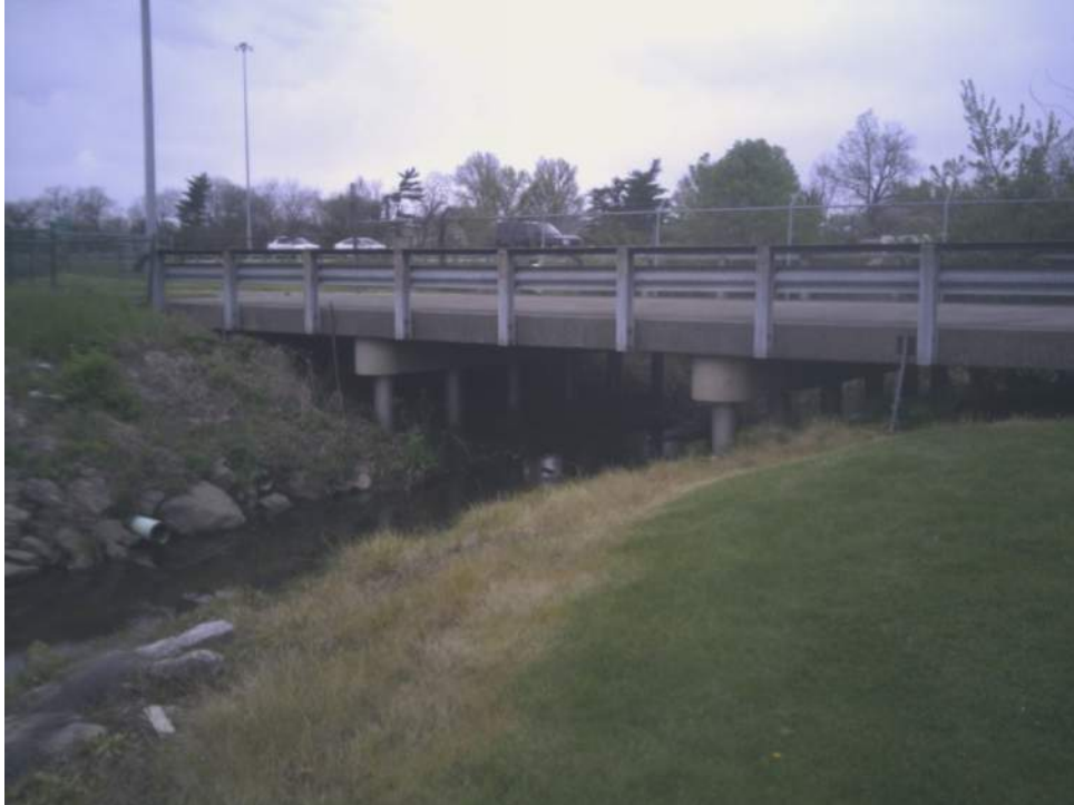
Figure 4. Existing Service Road Bridge (looking upstream)
