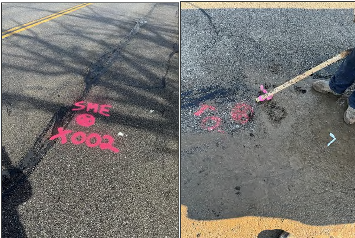
FIGURE NOS. 3 & 4: Before and after photographs of X-002-0-24.
