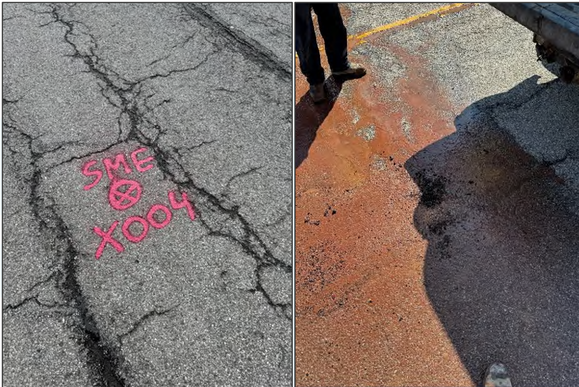
FIGURE NOS. 7 & 8: Before and after photographs of X-004-0-24.
