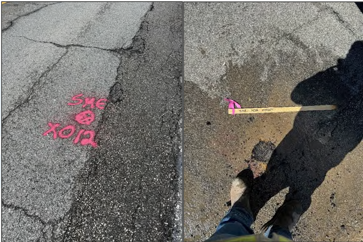
FIGURE NOS. 23 & 24: Before and after photographs of X-012-0-24.
