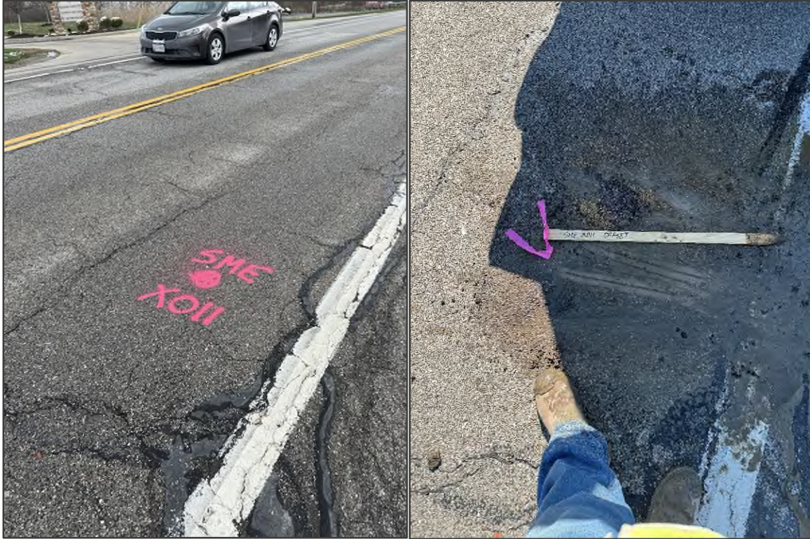
FIGURE NOS. 21 & 22: Before and after photographs of X-011-0-24.
