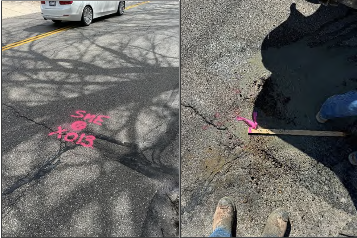
FIGURE NOS. 25 & 26: Before and after photographs of X-013-0-24.
