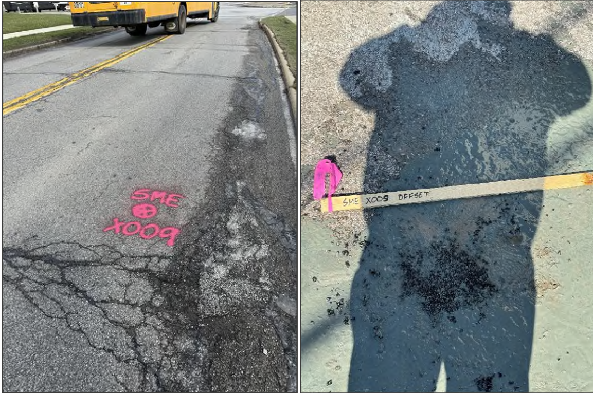
FIGURE NOS. 17 & 18: Before and after photographs of X-009-0-24.
