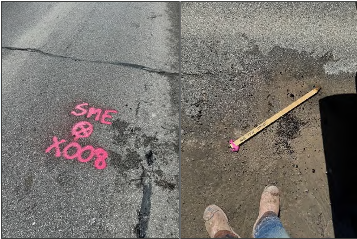
FIGURE NOS. 15 & 16: Before and after photographs of X-008-0-24.
