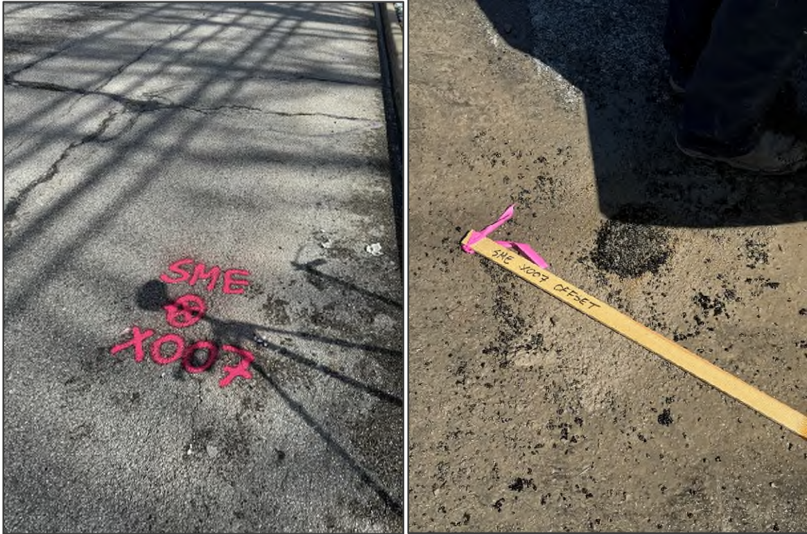
FIGURE NOS. 13 & 14: Before and after photographs of X-007-0-24.
