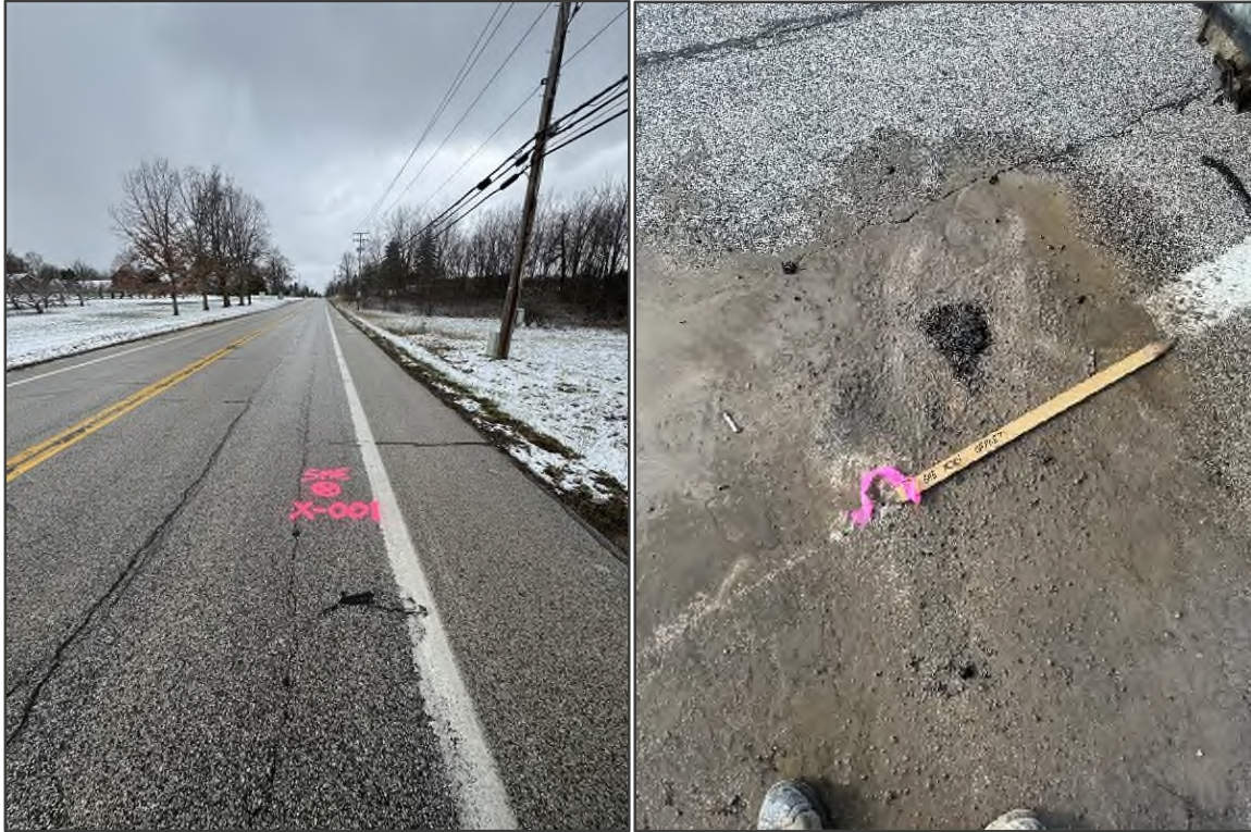
FIGURE NOS. 1 & 2: Before and after photographs of X-001-0-24.
