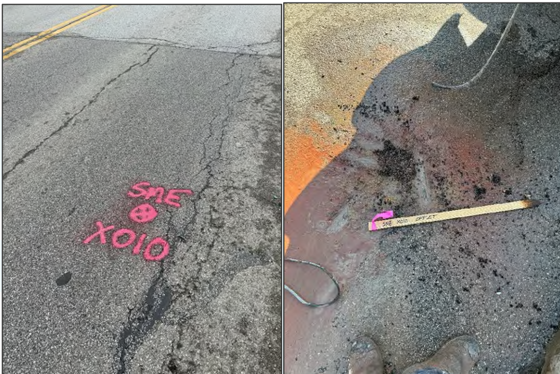
FIGURE NOS. 19 & 20: Before and after photographs of X-010-0-24.
