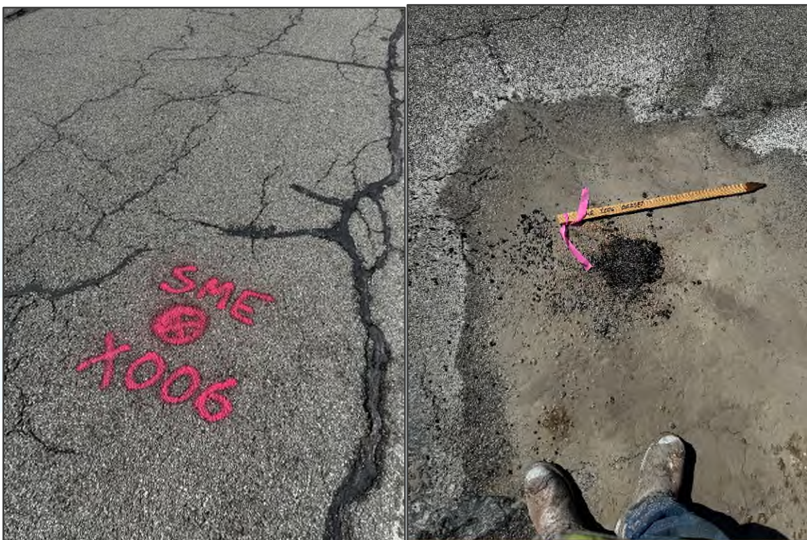
FIGURE NOS. 11 & 12: Before and after photographs of X-006-0-24.
