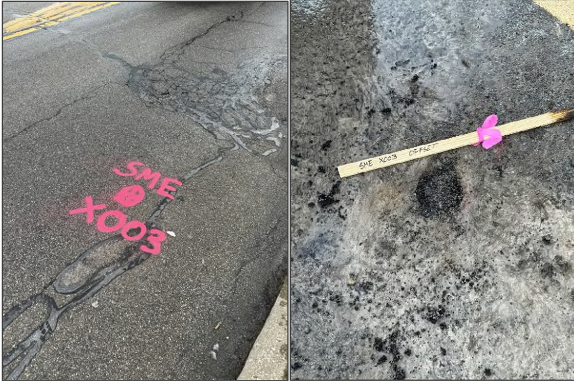
FIGURE NOS. 5 & 6: Before and after photographs of X-003-0-24.
