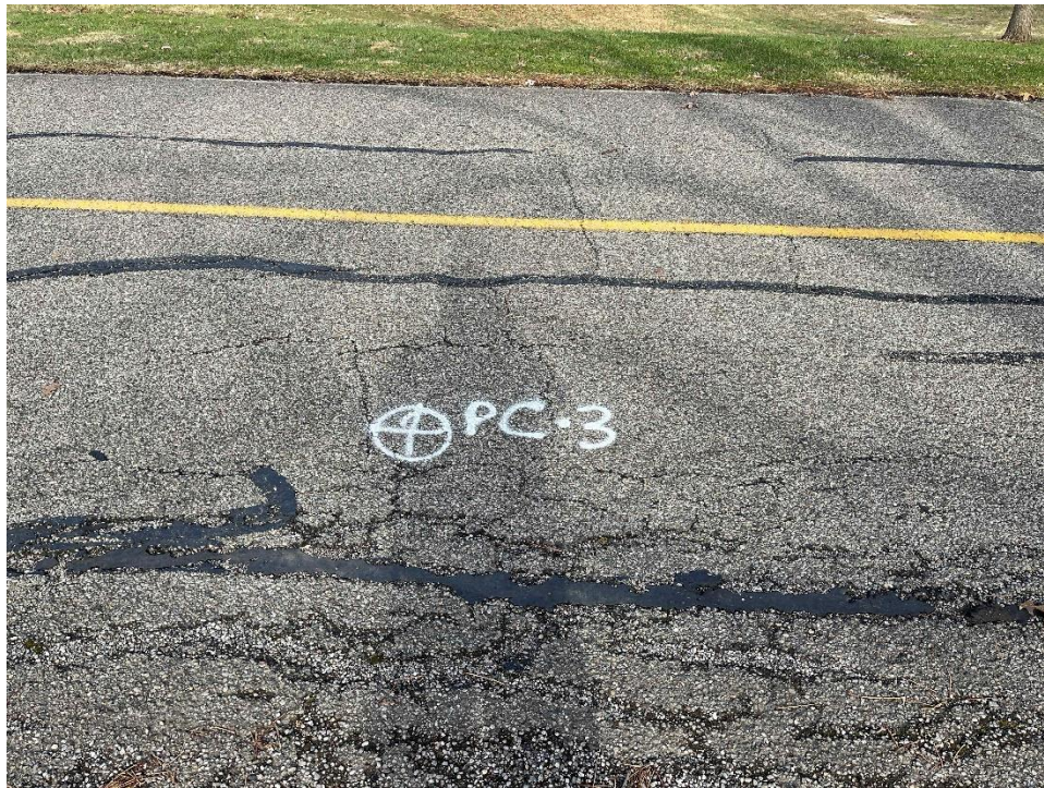
Site Photograph 3. Pavement Core PC-3 (photograph taken December 1, 2022).
