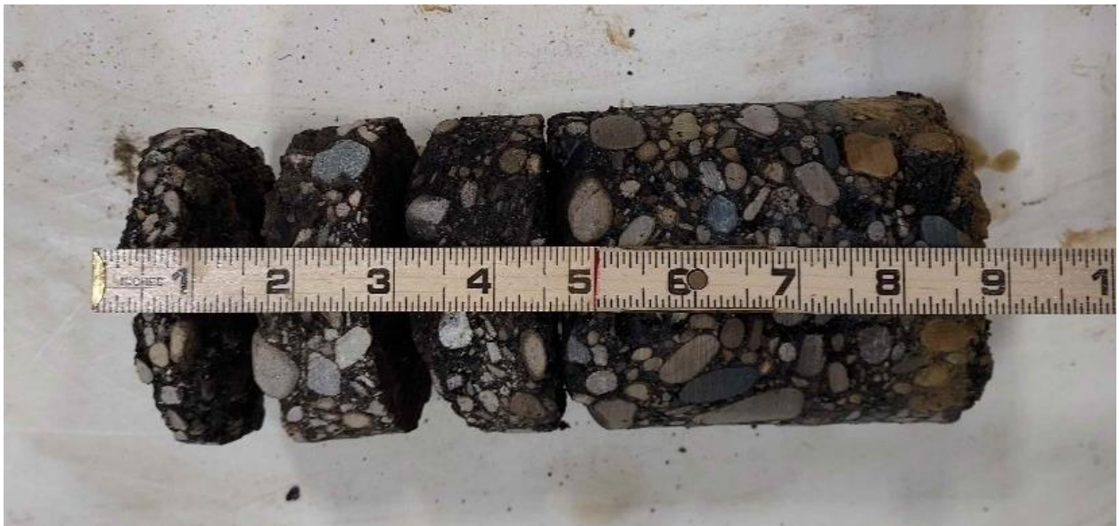
Pavement Core Photograph 4. Pavement Core PC-4.
