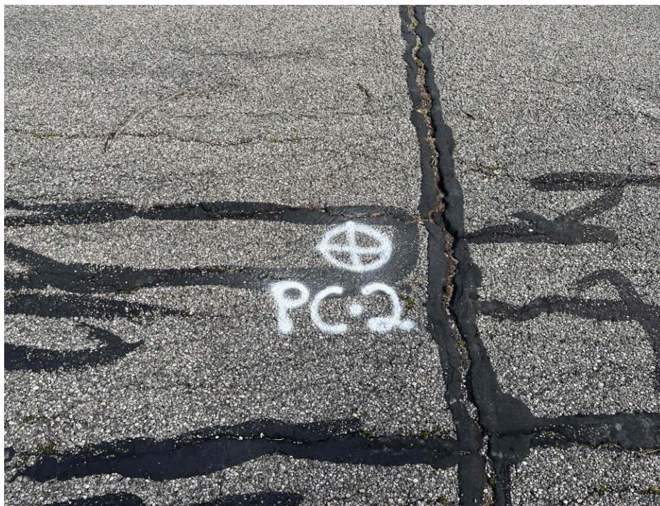
Site Photograph 2. Pavement Core PC-2 (photograph taken December 1, 2022).
