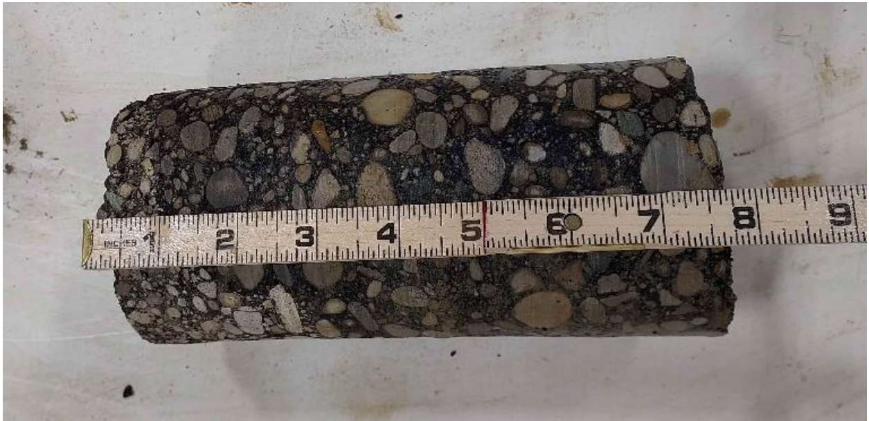
Pavement Core Photograph 3. Pavement Core PC-3.
