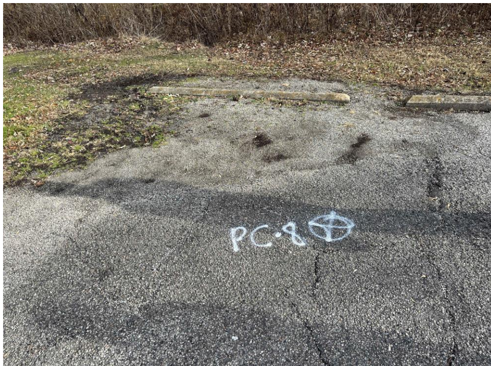
Site Photograph 8. Pavement Core PC-8 (photograph taken December 1, 2022).
