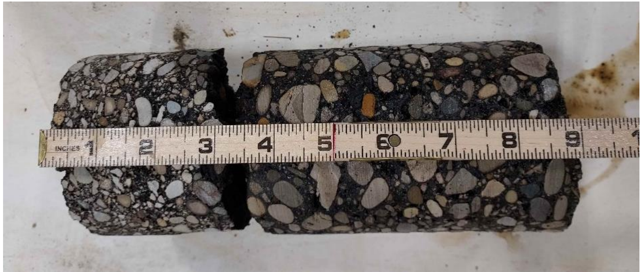
Pavement Core Photograph 7. Pavement Core PC-7.
