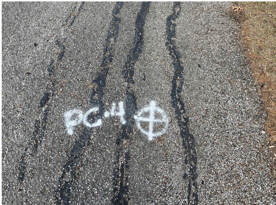
Site Photograph 4. Pavement Core PC-4 (photograph taken December 1, 2022).
