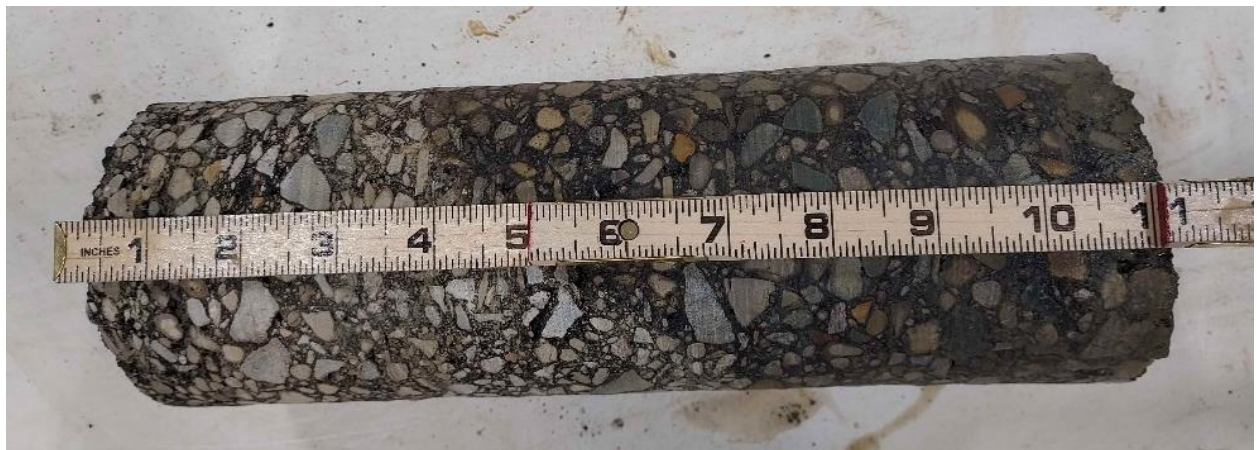
Pavement Core Photograph 8. Pavement Core PC-8.
