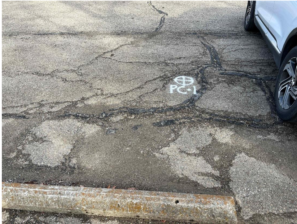
Site Photograph 1. Pavement Core PC-1 (photograph taken December 1, 2022).
