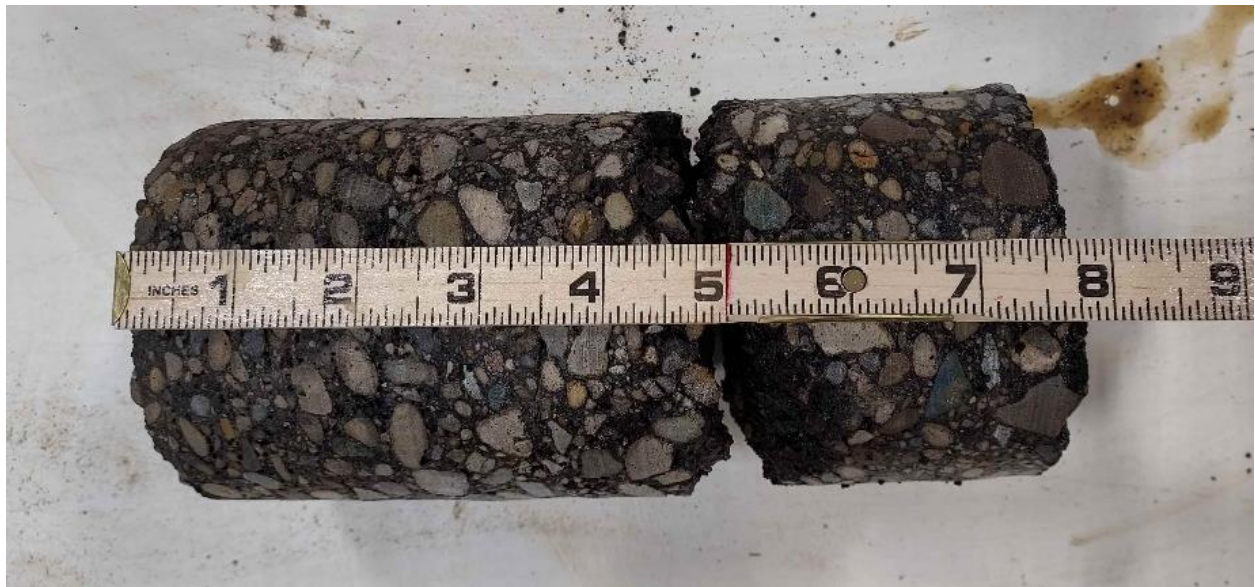
Pavement Core Photograph 5. Pavement Core PC-5.
