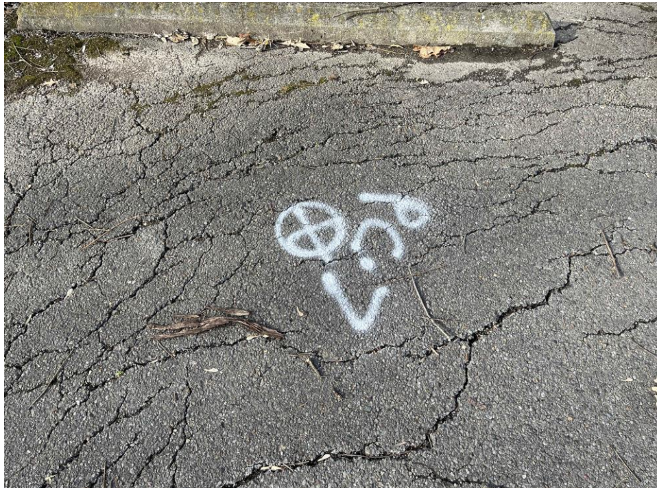
Site Photograph 7. Pavement Core PC-7 (photograph taken December 1, 2022).
