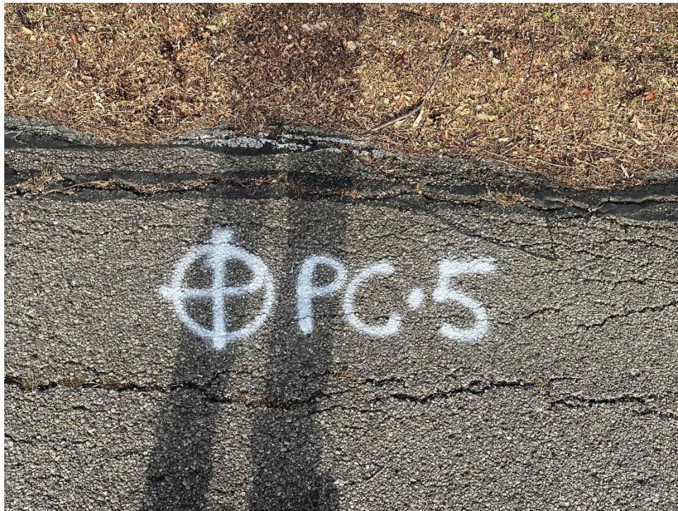
Site Photograph 5. Pavement Core PC-5 (photograph taken December 1, 2022).
