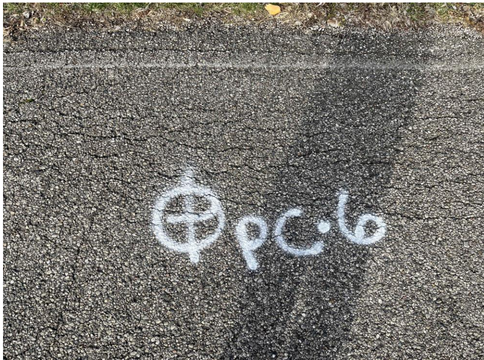
Site Photograph 6. Pavement Core PC-6 (photograph taken December 1, 2022).
