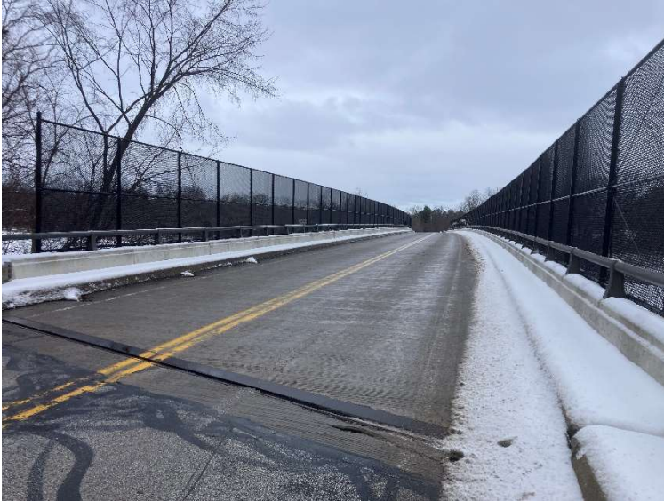
PHOTO 1 View of bridge LAK-90-11.51, facing north.
