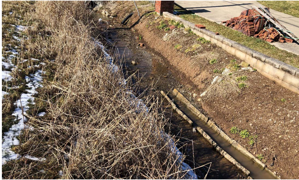
Photograph 1: Toe of Southeastern Embankment and Drainage Ditch
