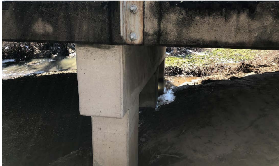
Photograph 3: Western Spill-through Slope
