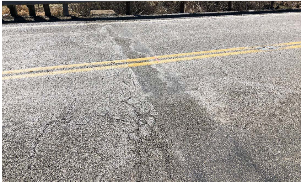
Photograph 7: Overall Condition of Asphalt Wearing Course
