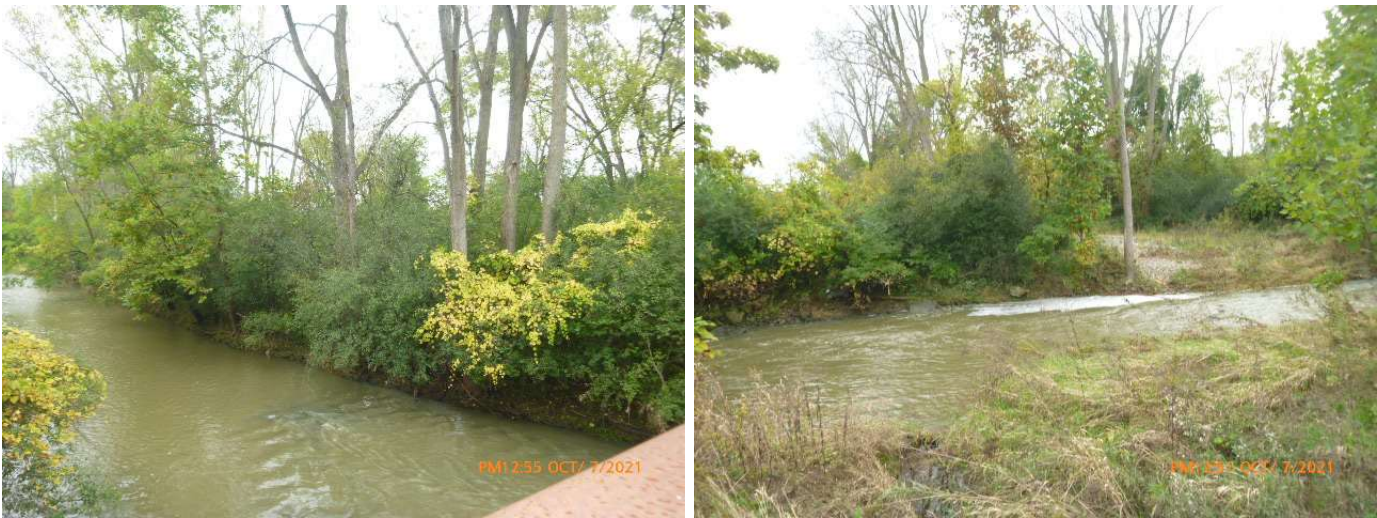
Fig. 04. Upstream US-23 (left), Downstream (right)
