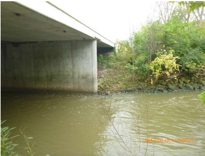
Fig. 10 Upstream View of US 23 Northbound Bridge
