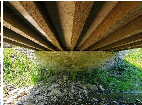
Facing West Abutment
