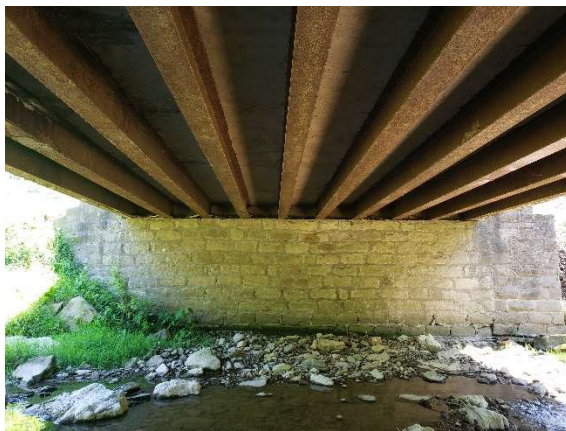
Facing East Abutment
