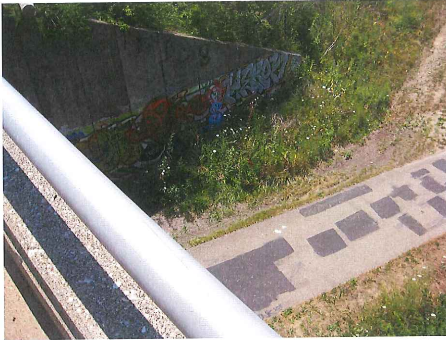
Photograph 7: Bridge MOT-CR-074-0.65, West Side of Bridge Facing Down, Southwest
