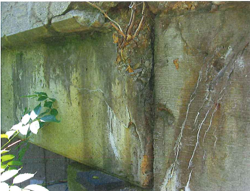
Photograph 2: Bridge MOT-CR-074-0.65, Tar @ Joints on Bike Path Side, Ends of Bridge
