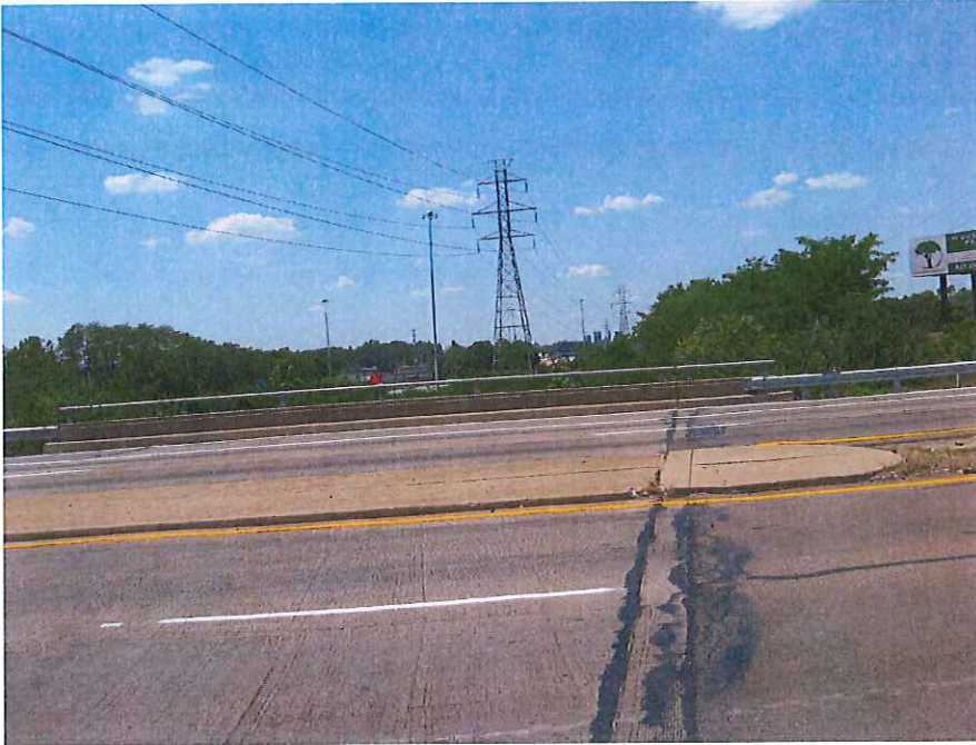
Photograph 3: Bridge MOT-CR-074-0.65, Top of Bridge Facing West
