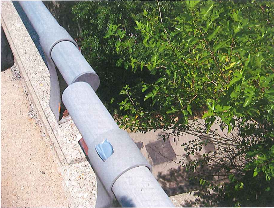
Photograph 1: Bridge MOT-CR-074-0.65, Facing Down Toward Bike Path, Northeast
