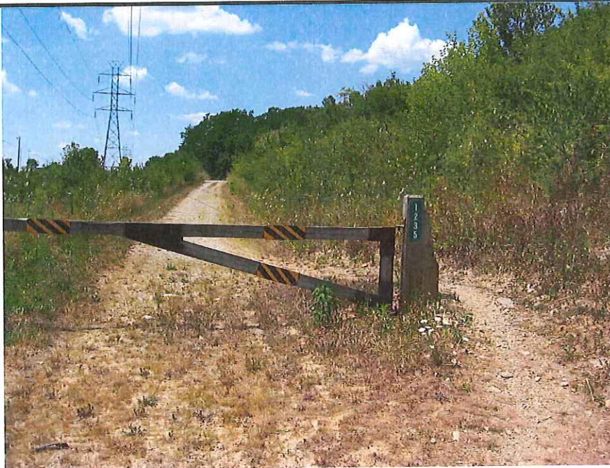
Photograph 8: Bridge MOT-CR-074-0.65, Locked Access Road at Spinning Road
