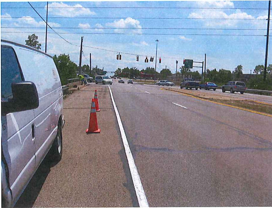
Photograph 5: Bridge MOT-CR-074-0.65, East Side of Roadway Facing South
