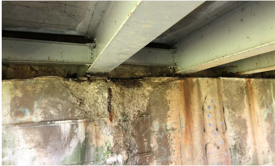
Photograph 4: Large Crack in Southeastern Abutment
