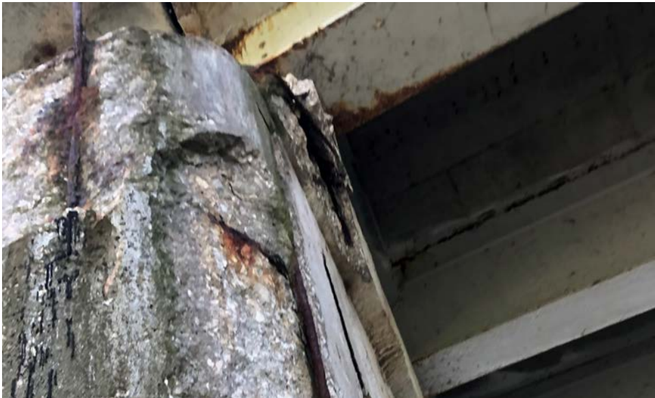
Photograph 6: Spalling and Exposed Rebar at Eastern End of Pier
