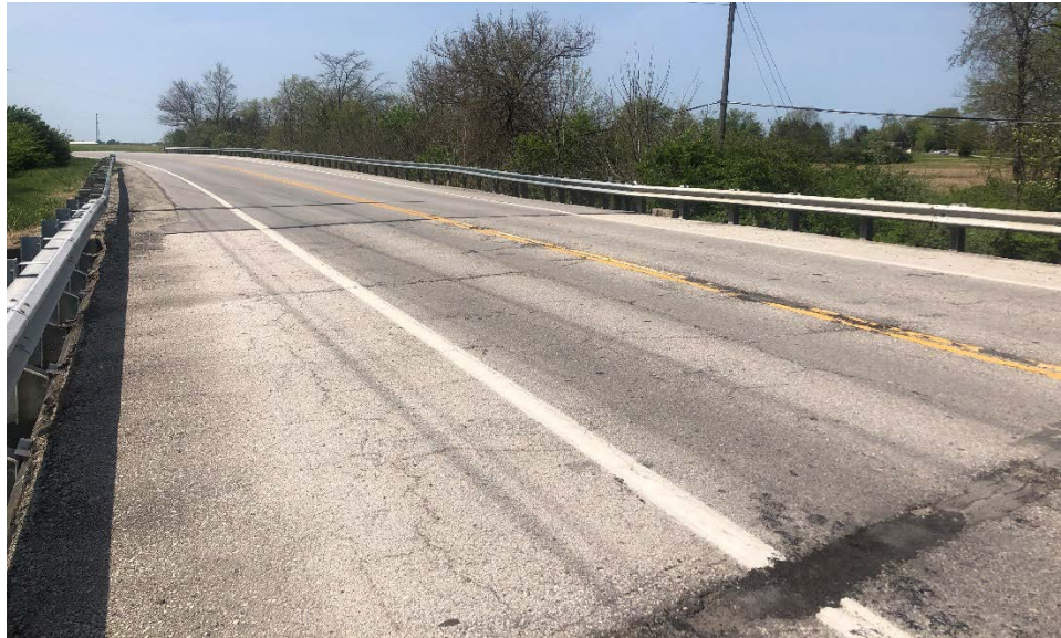
Photograph 9: Asphalt Wearing Course
