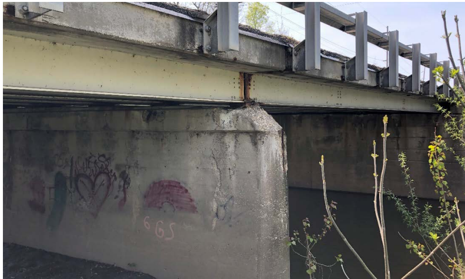
Photograph 2: Corrosion and Section Loss at Mid-Span Beam Ends and Stringers
