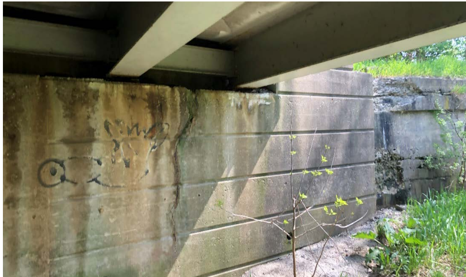
Photograph 4: Large Crack in Southeastern Abutment
