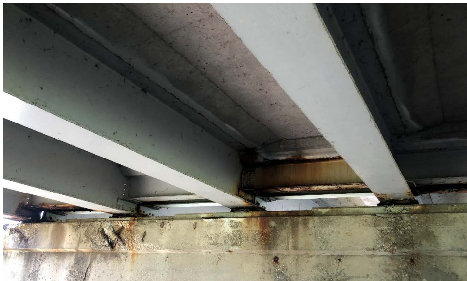
Photograph 2: Corrosion and Section Loss at Mid-Span Beam Ends and Stringers
