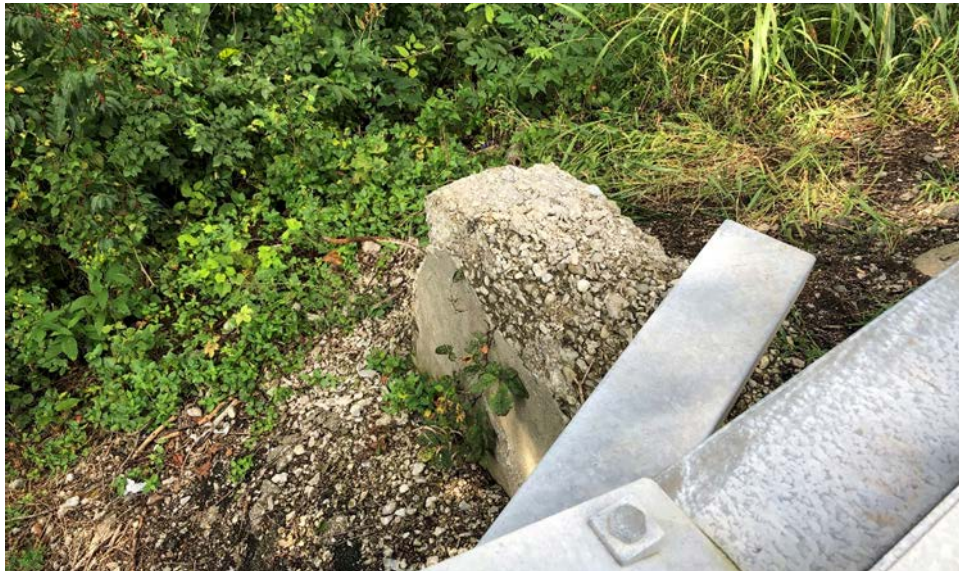
Photograph 6: Observed Deterioration of Northwestern Wingwall
