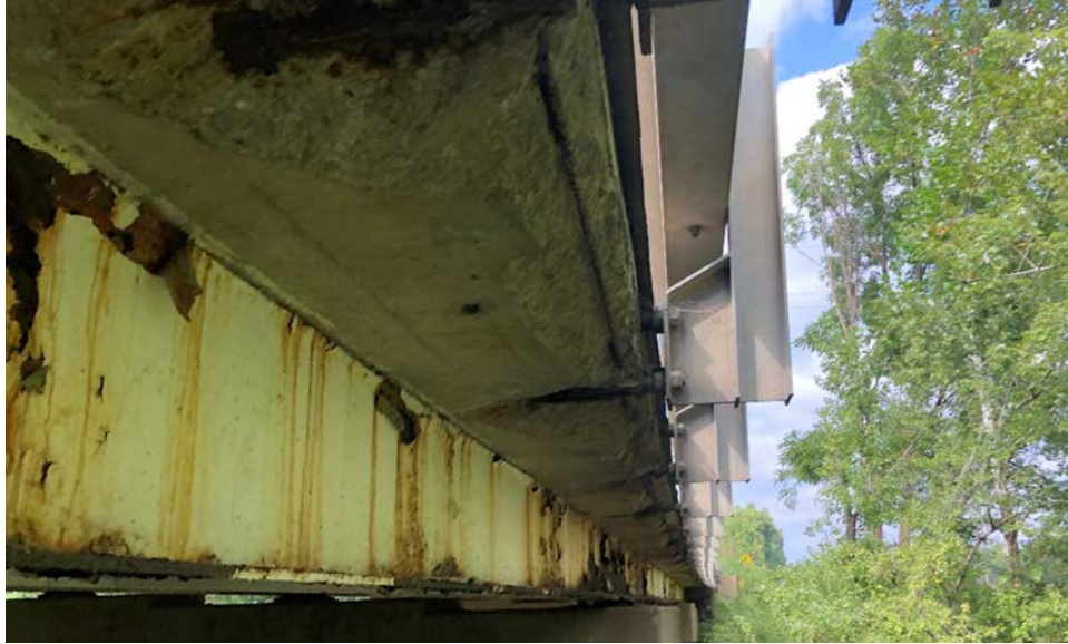
Photograph 6: Observed Deterioration of Northwestern Wingwall
