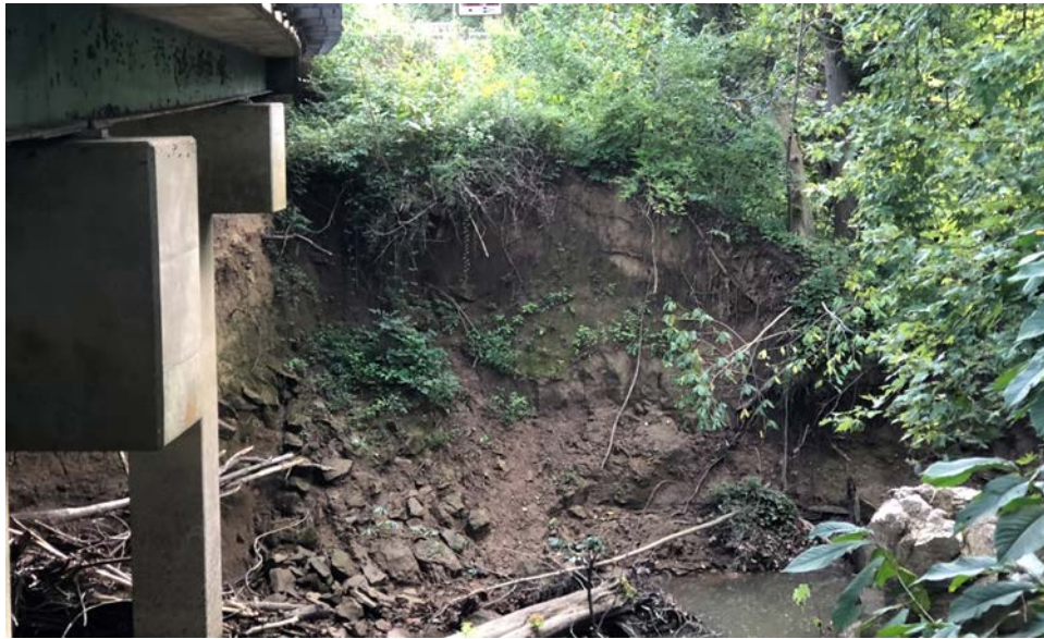
Photograph 3: Western End of Southern Spill Through Slope
