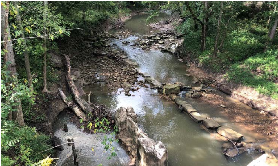
Photograph 1: Original Bridge Pier Remains West of Current Bridge
