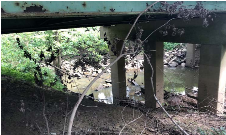
Photograph 2: Spill Through Slopes
