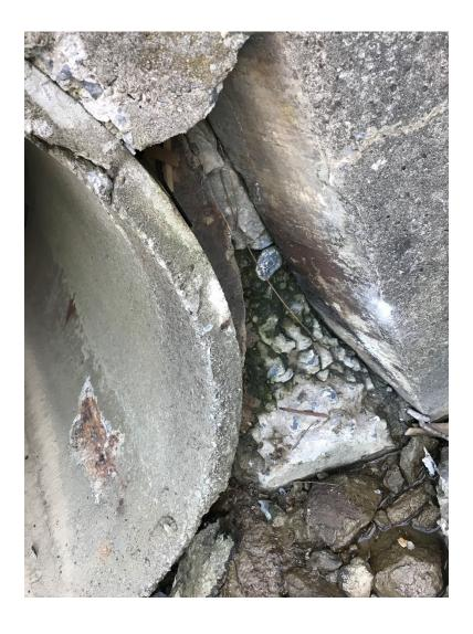
Photograph 2 – View of Culvert Pipe Inlet- 10% Chrysotile Asbestos (B004)
