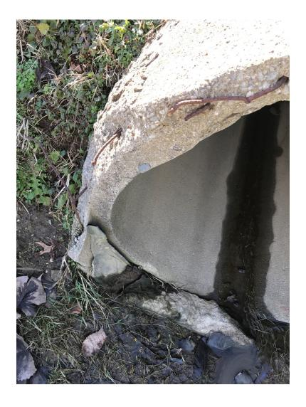
Photograph 3 – View of Culvert Pipe Outlet- 10% Chrysotile Asbestos (B006)
