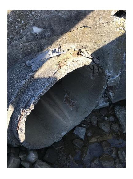
Photograph 1 – View of Culvert Pipe Inlet- 10% Chrysotile Asbestos (B001)
