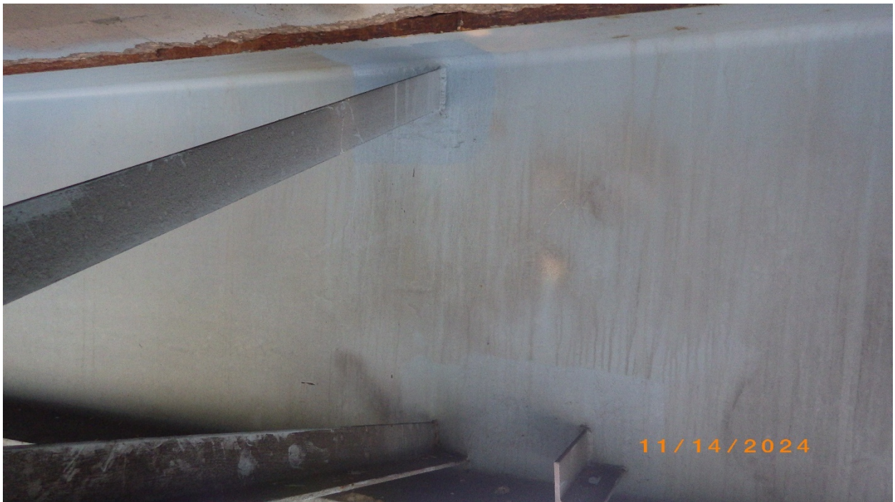
Photo # 33 – Crossframe 5 at Beam 2
