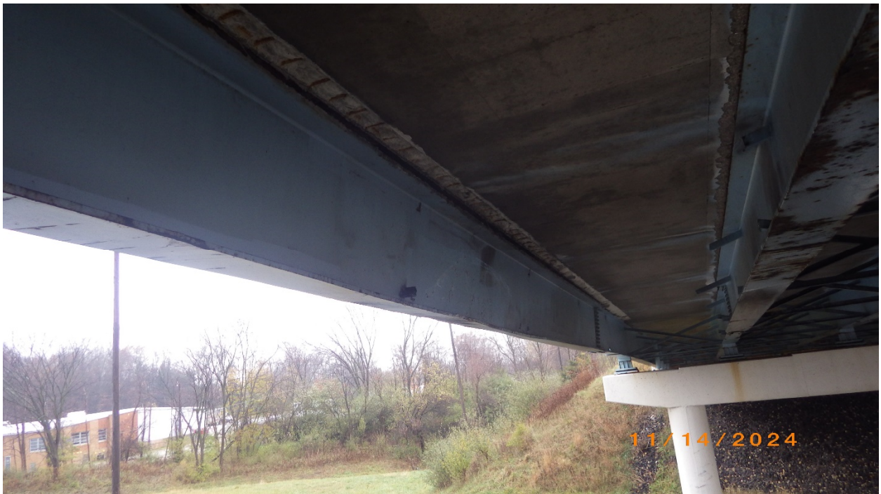
Photo # 10 - Bay 1, looking North from Crossframe 3, following removal of Crossframes 3-7
