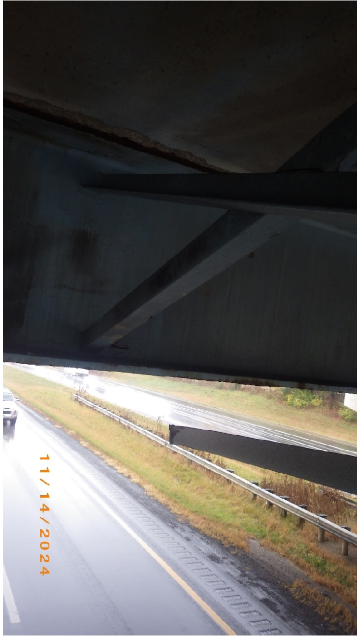
Photo # 29 – Crossframe 4 at Beam 2
