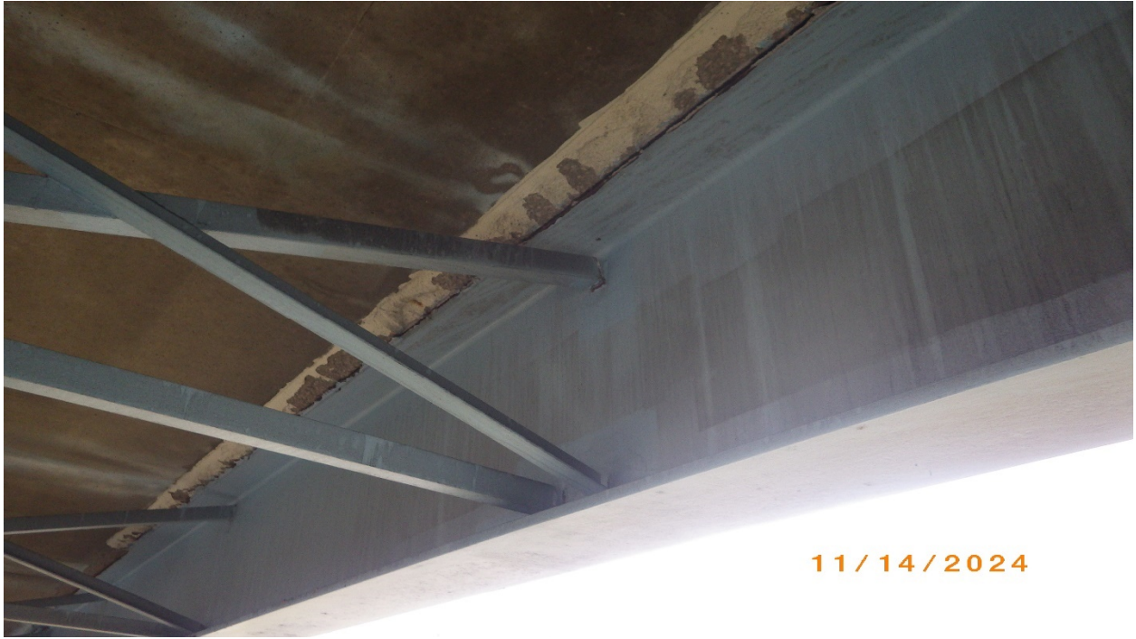
Photo # 24 – Crossframe 2 at Beam 1
