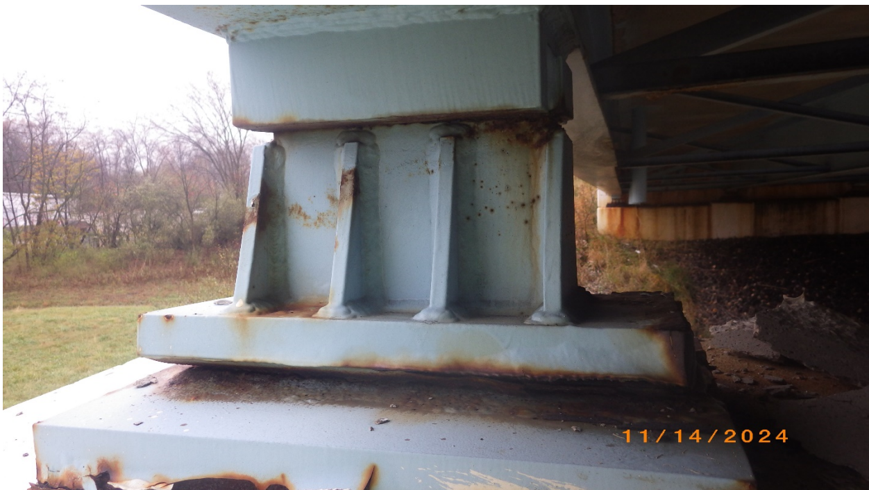
Photo # 16 – Bearing 1, Pier 3
