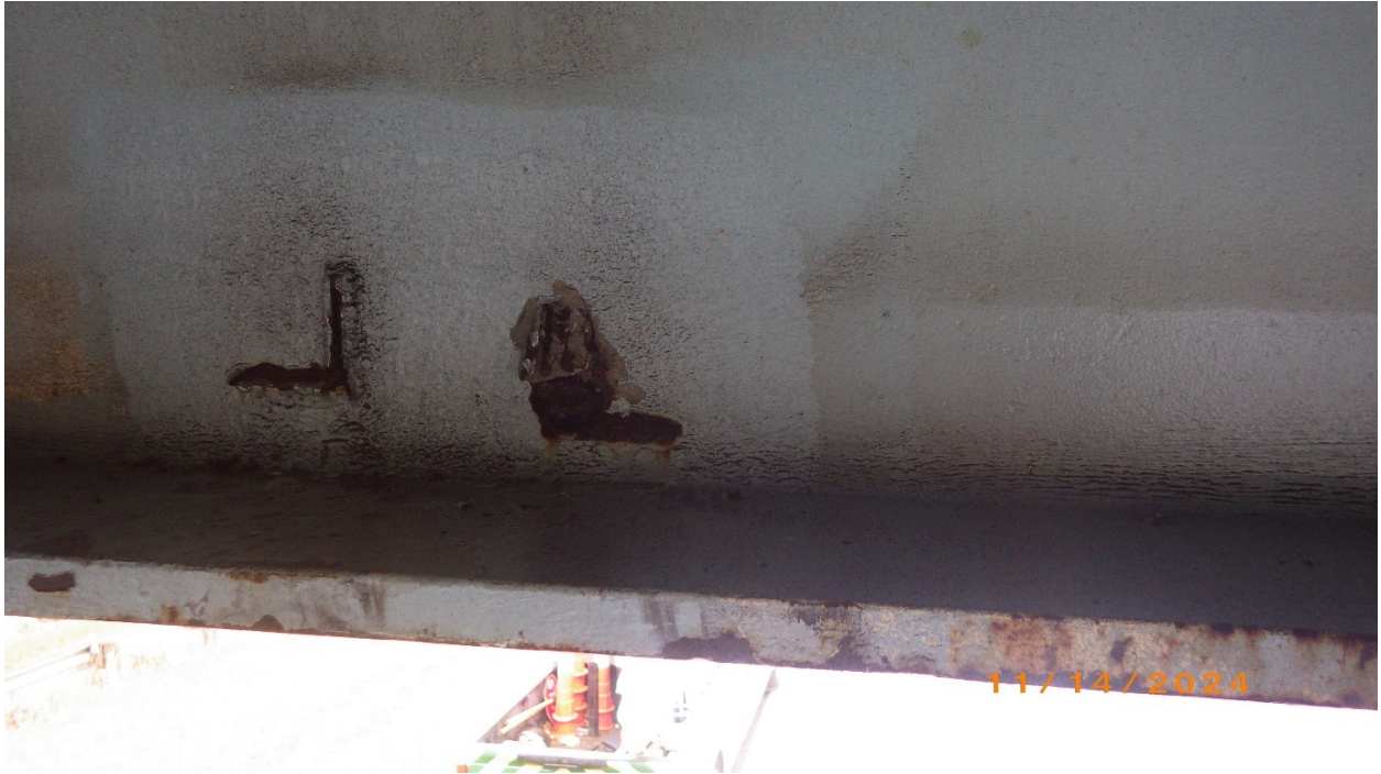
Photo # 26 – Crossframe 3 at Beam 1, lower welds
