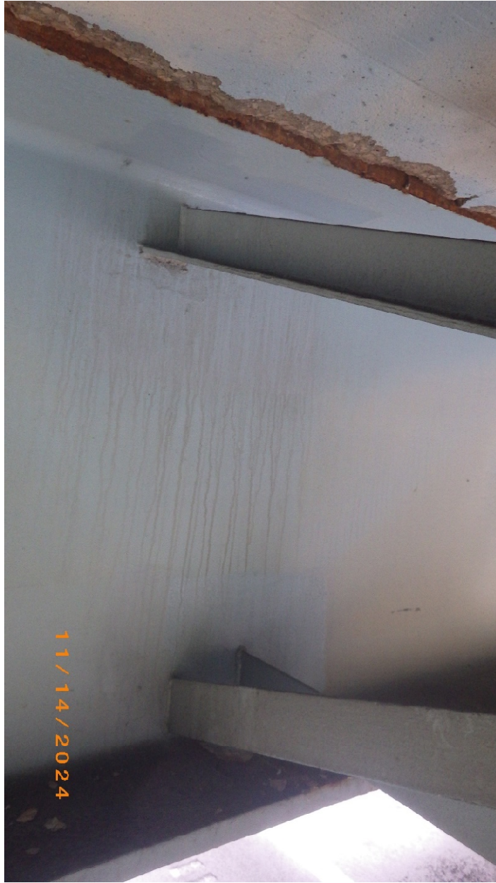
Photo # 35 – Crossframe 6 at Beam 2
