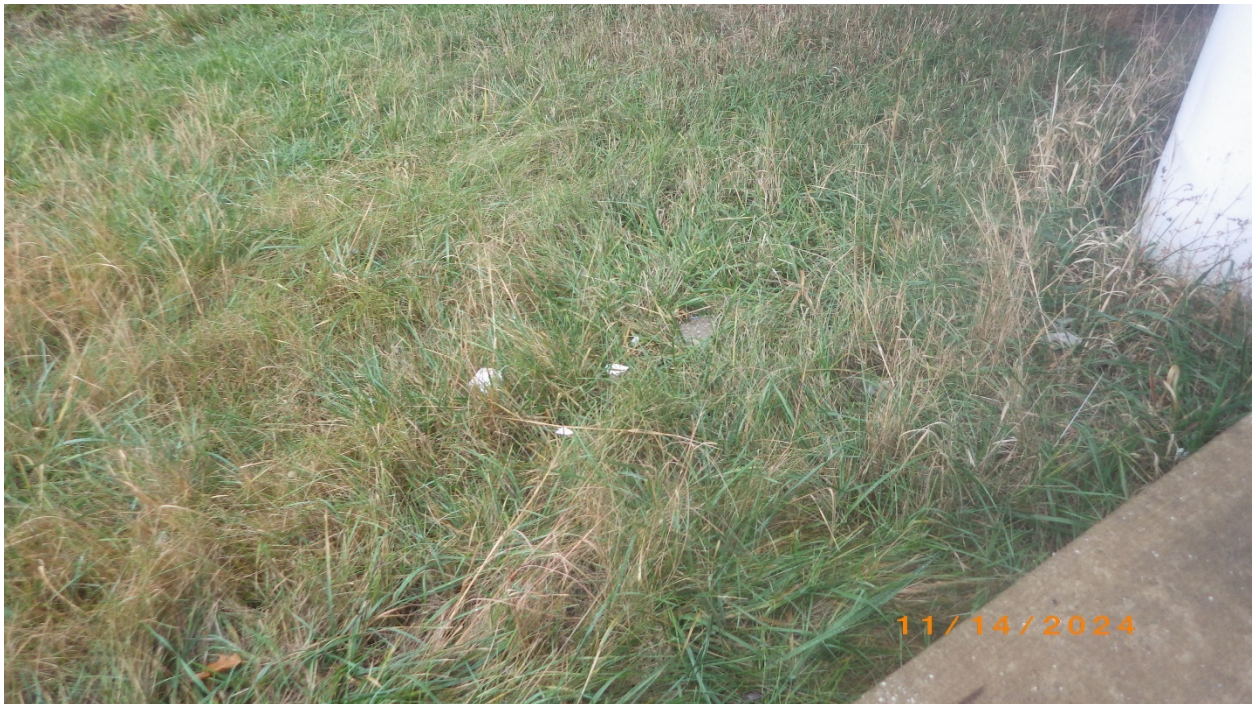
Photo # 20 – Fresh spalling on shoulder, North side of Westbound roadway
