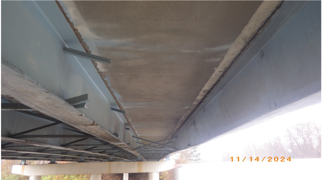
Photo # 9 - Bay 1, looking South from Crossframe 7 following removal of Crossframes 4-7
