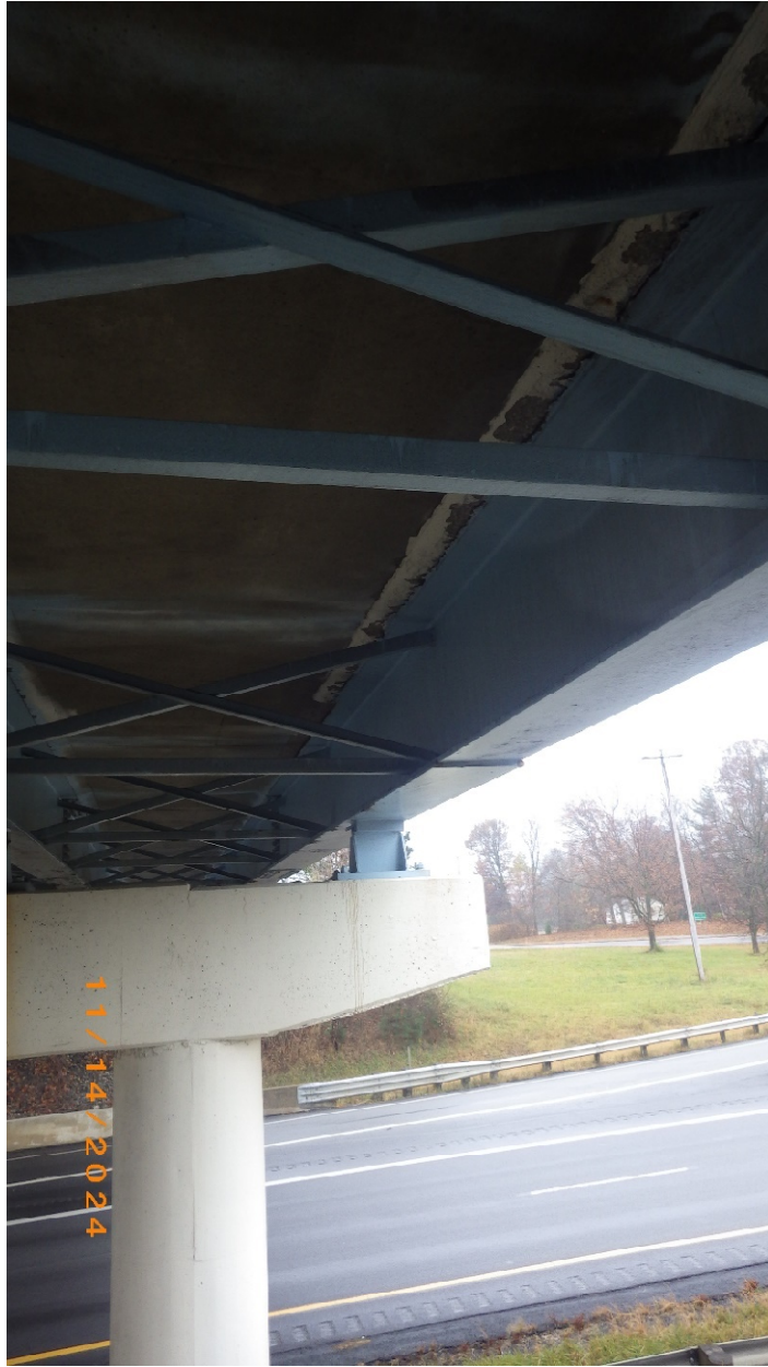
Photo # 23 – Crossframe 1 & 2, looking south
