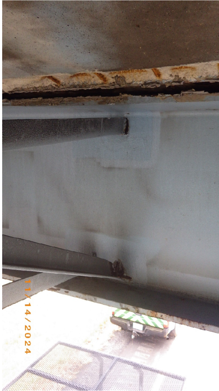
Photo # 25 – Crossframe 3 at Beam 1
