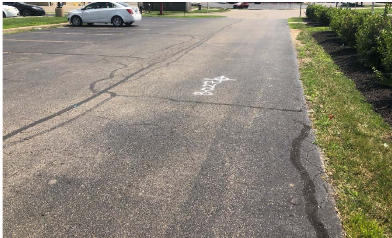
Photograph 5: Overall Pavement condition of Parking Lot
