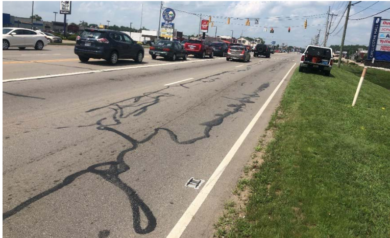
Photograph 3: Overall Pavement condition of N Bridge St Between
