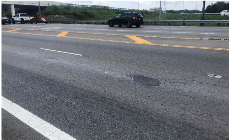
Photograph 1: Overall Pavement Condition of North Bridge Street near US-35
