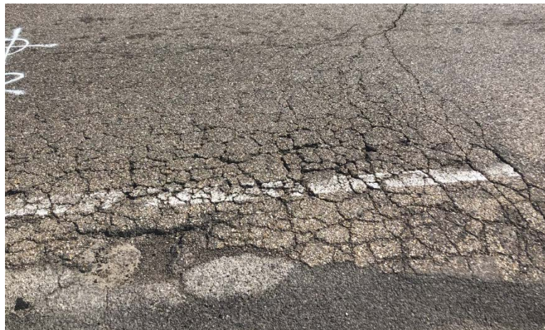
Photograph 1: Patching and cracking along edge of existing CR-550
