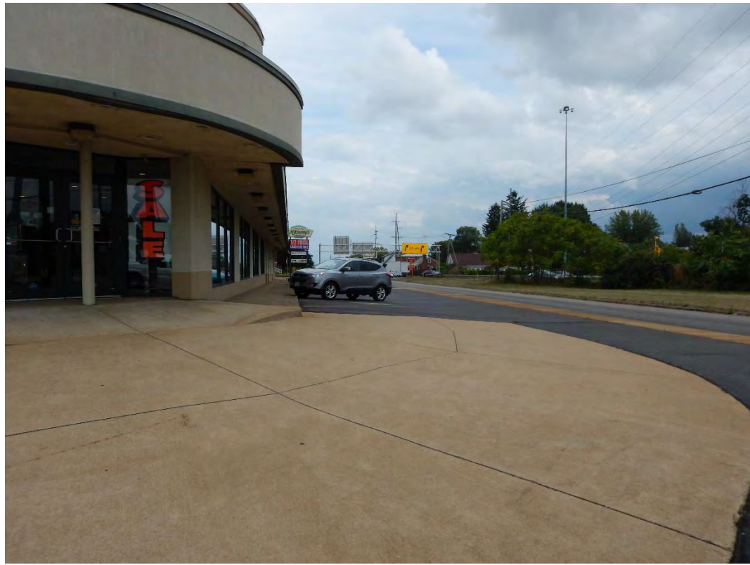
Photo 6 Site W 1001 30 th Street NE Canton, OH 44714 Standing at corner of 30 th Street and Martindale Road looking E along the South side of McKinney's Outlet building
