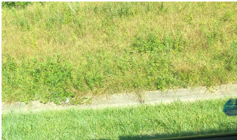
Photograph 4: Paved drainage swale between Shade Road and Ira Road
