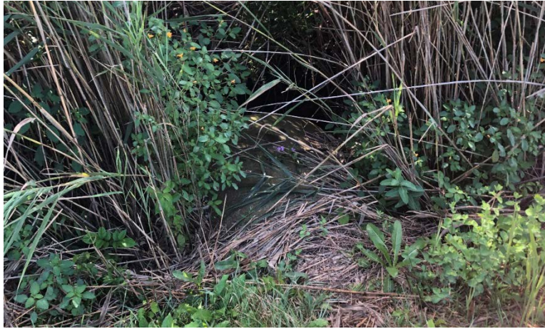
Photograph 3: Culvert directing drainage from median to east of IR-77 NB
