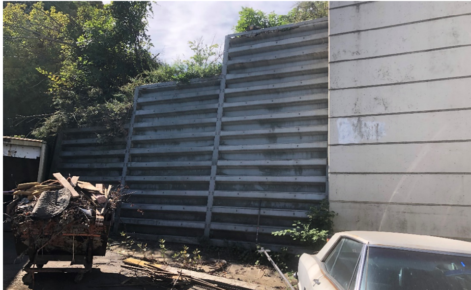
Photograph 4: Steel Retaining Wall at Southeastern Corner of Bridge
