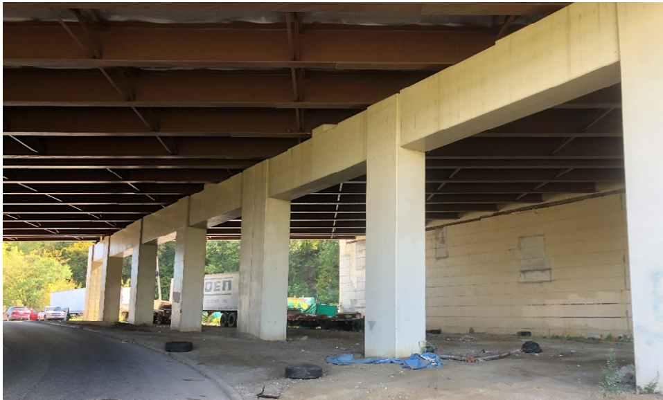
Photograph 2: Beacon Street Bridge
