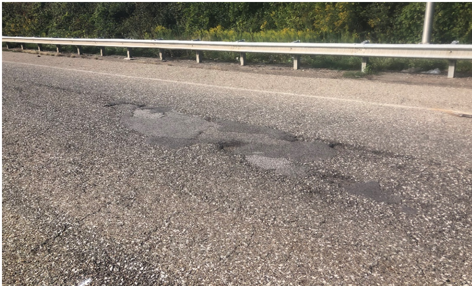
Photograph 6: Overall Pavement Condition of Ramps
