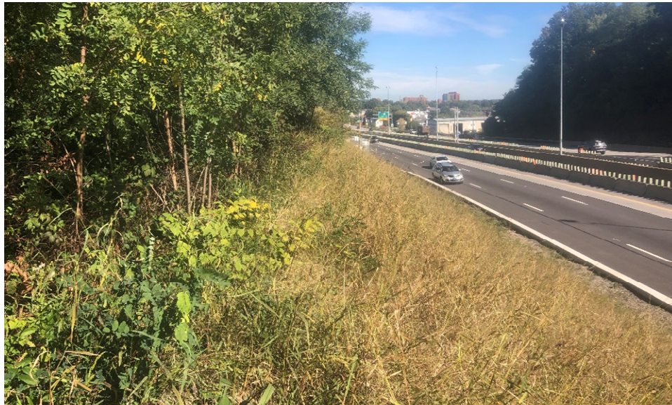
Photograph 1: Existing Embankment in the Area of the Proposed Retaining Wall
