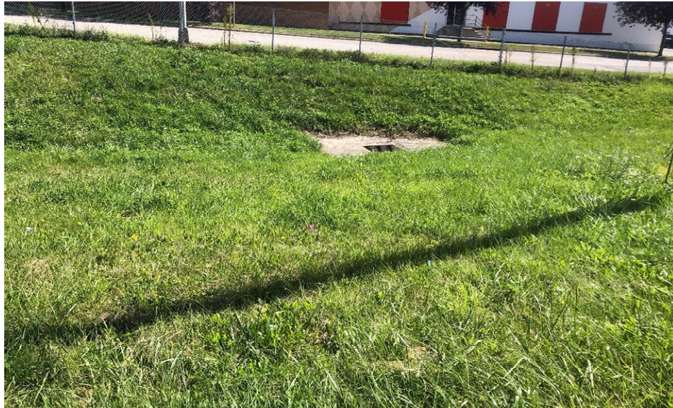
Photograph 7: Example of Drainage Ditches and Drainage Basin
