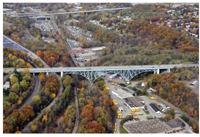
ramp from Perkins Street will essentially be extended across the bridge to become the exit ramp for the Glenwood Avenue interchange. For SR-8 south, the southbound entrance ramp from Glenwood Avenue will extend across the bridge to the exit ramp for the Perkins Street interchange.
