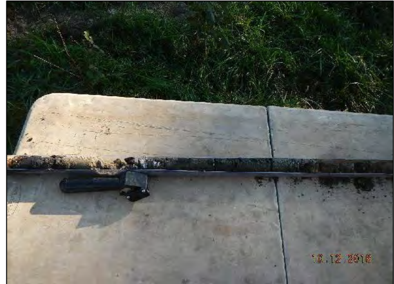
Photo 2 – View of soil profile at EB-1 (0-5' below ground surface [bgs]). See soil boring logs for soil profile description.
