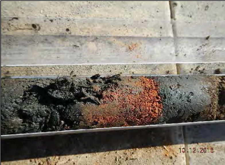
Photo 17 - Close up view of debris materials at EB-4 (brick and wood fragments).
