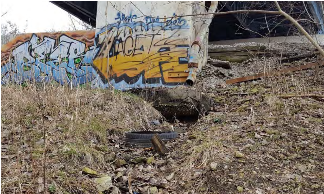
Photograph 1: Sign of erosion at storm sewer outlet under south side of existing bridge (1 of 2)
