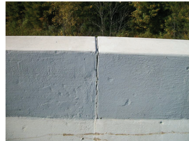
Photograph 2. SR 250 ramp bridge over I-77 and East Stone Creek, concrete barrier caulk (Sample 1232R-01).
