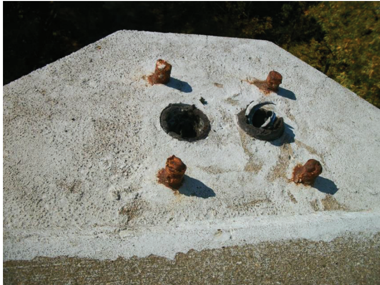
Photograph 4. SR 250 ramp bridge over I-77 and East Stone Creek, light pole conduit insulation (Sample 1232-03).
