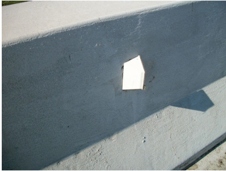
Photograph 3. SR 250 ramp bridge over I-77 and East Stone Creek, reflector glue (Sample 1232R-02).
