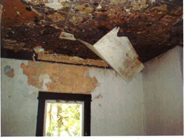
Second floor, Apartment ceiling
