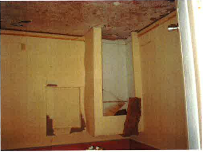
Second floor, Apartment
