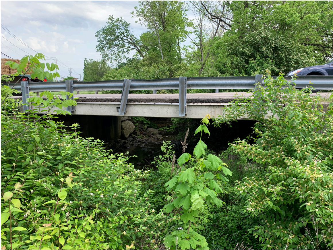
Upstream Face STA–Spangler Street
