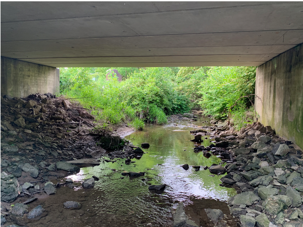
Downstream Face STA–Spangler Street
