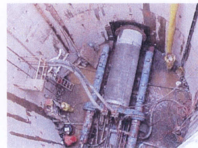
Microtunneling from a caisson
