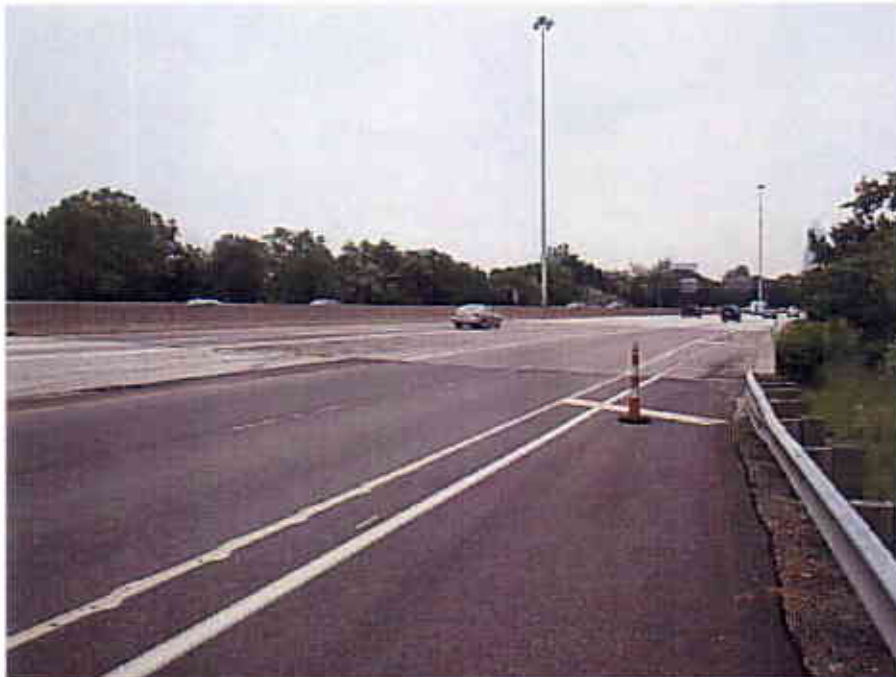
Photograph 46 View Looking North at the Top of the East Bound Lanes of the Interstate 90 Bridge over Starkweather Avenue (CUY-90-1490R)
