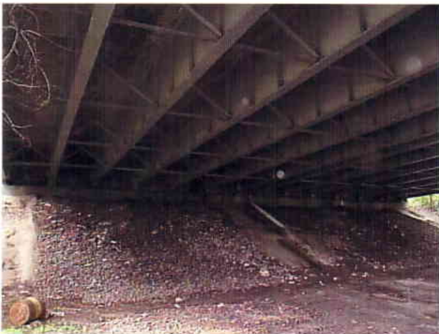
Photograph 14 View Looking West at the Underside of the East and West Bound Lanes of the Interstate 90 Bridge over Ramps E-10 and E-8 (CUY-90-1640)
