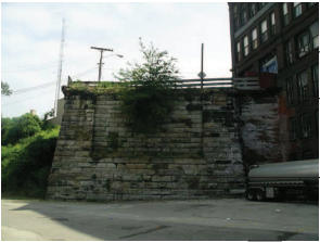
STONE ABUTMENT WALL / BROADWAY MILLS BUILDING FOUND
