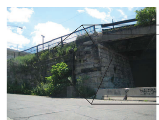
STONE ABUTMENT WALL
