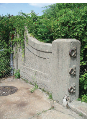
EAGLE AVE CONCRETE ABUTMENT WALL
