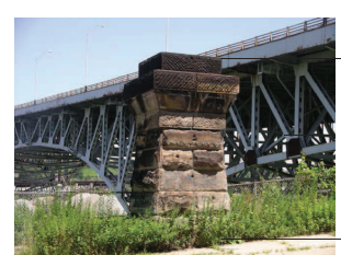
STONE PIER COLUMNS
