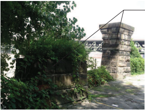
STONE PIER COLUMNS
