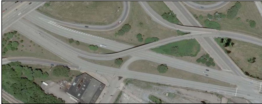
Figure 4.2 NB Ontario between E.9 th Street and Carnegie
