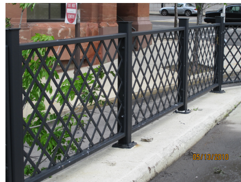
ORNAMENTAL RAILING PHOTO FROM EAST END OF DETROIT SUPERIOR BRIDGE
