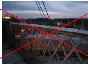
FENCING ON STONE ABUTMENT WALL
