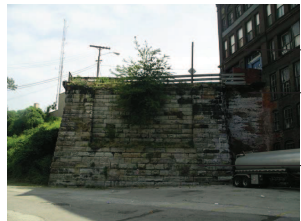
STONE ABUTMENT WALL / BROADWAY MILLS BUILDING FOUND
