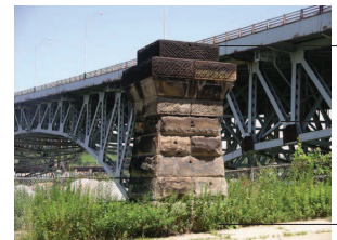
STONE PIER COLUMNS
