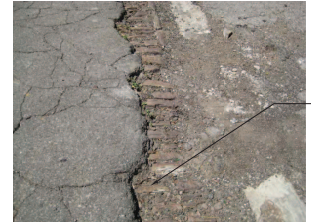
PAVERS ON UNIVERSITY DRIVE
