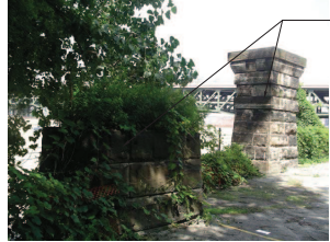
STONE PIER COLUMNS
