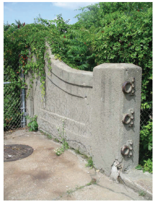
EAGLE AVE CONCRETE ABUTMENT WALL
