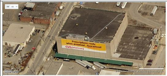
Watson describes this building as being "of unique design" with 12-inch concrete outer walls and 16-inch concrete bearing inner walls with 16-inch of ground cork between them (as insulation). This building has some decorative details, but fewer than the Distribution Terminal Warehouse, designed by Watson.
