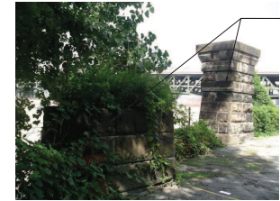
STONE PIER COLUMNS
