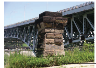
STONE PIER COLUMNS
