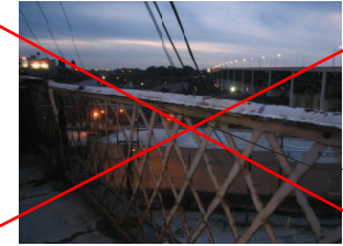
FENCING ON STONE ABUTMENT WALL
