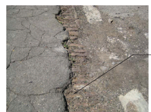
PAVERS ON UNIVERSITY DRIVE
