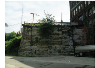
STONE ABUTMENT WALL / BROADWAY MILLS BUILDING FOUND
