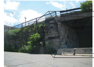
STONE ABUTMENT WALL
