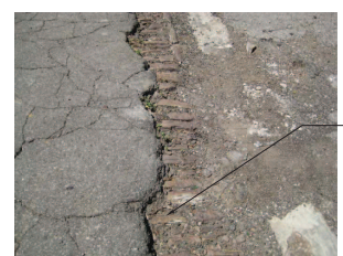
PAVERS ON UNIVERSITY DRIVE
