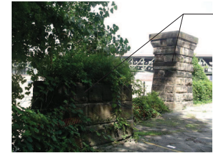
STONE PIER COLUMNS
