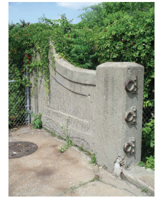
EAGLE AVE CONCRETE ABUTMENT WALL
