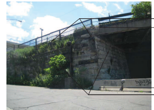
STONE ABUTMENT WALL
