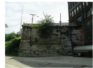
STONE ABUTMENT WALL / BROADWAY MILLS BUILDING FOUND
