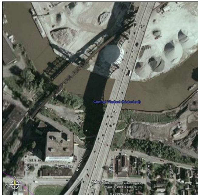
Aerial of Existing Structure over Cuyahoga River
